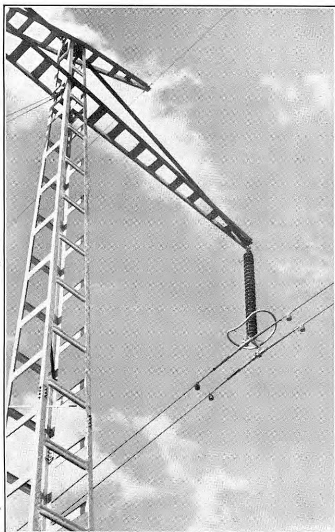
FIG. 13. DOUBLE CONDUCTOR SUPPORTED BY SINGLE INSULATOR STRING.
