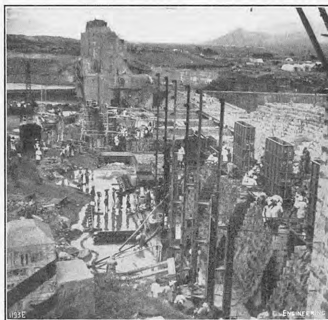
FIG. 10. ERECTION OF SLUICE GATES.
