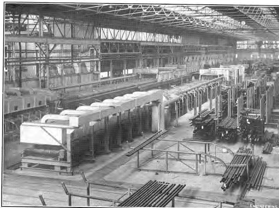
FIG. 15. NORMALISING FURNACE.
