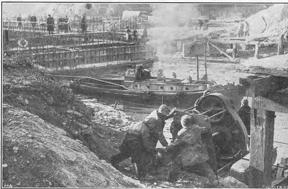
FIG. 1. PARTLY-CONSTRUCTED INTAKE LEAVING DRY DOCK.
