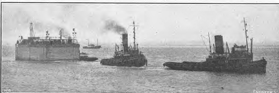
FIG. 3. TOWING COMPLETED INTAKE FROM TILBURY TO CORYTON.
