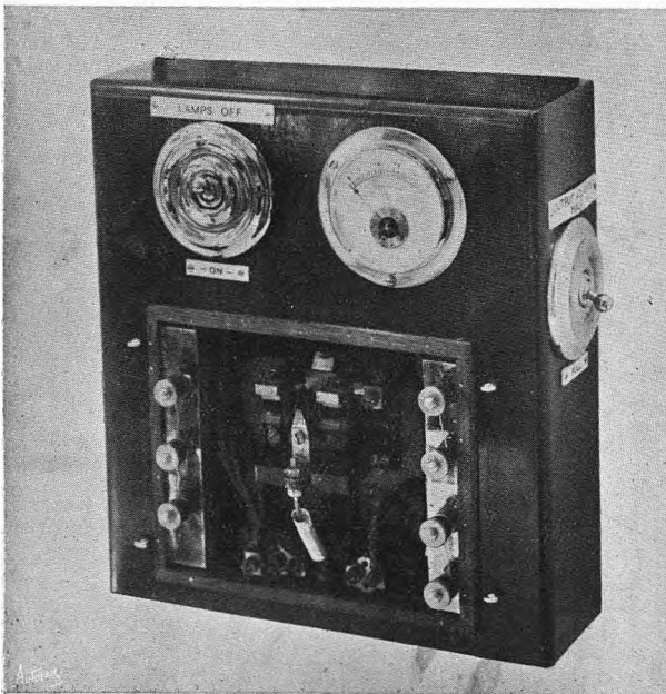
The C.A.V. switch-board with cover removed, showing cut-out.
