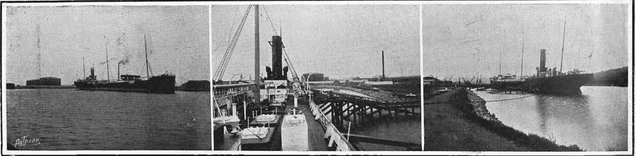
A good idea of the shipping facilities for petrol at Portishead may be obtained from the above illustrations, which show one of the Company's tank steamers at her moorings.
