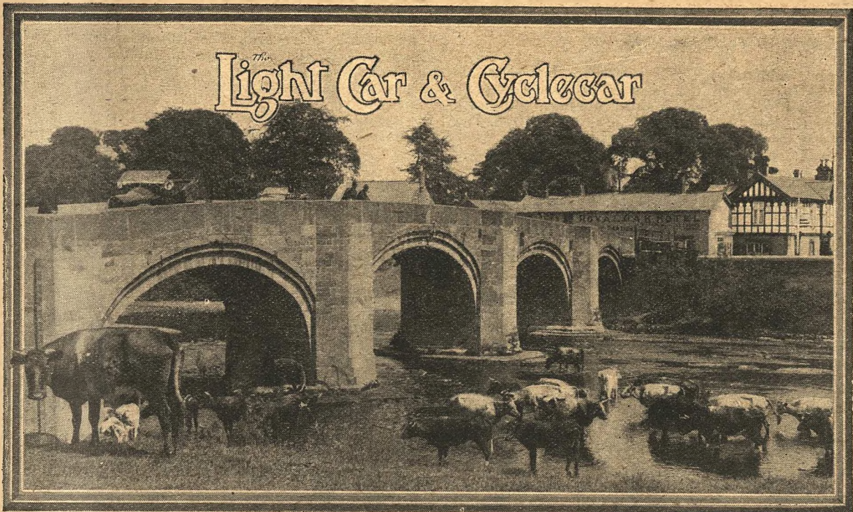
Crossing the bridge at Bangor.
