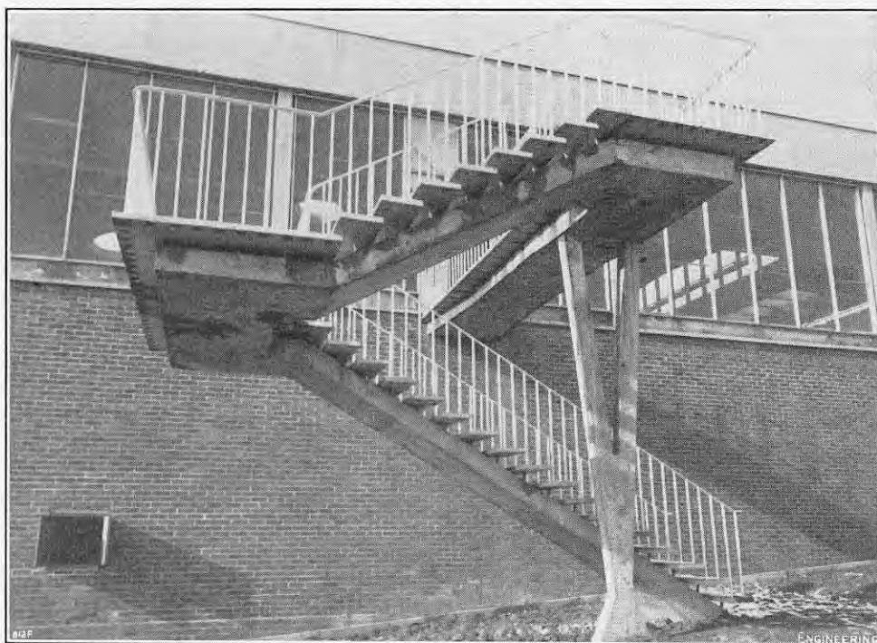
FIG. 10. ESCAPE STAIRWAY OF REINFORCED CONCRETE.
