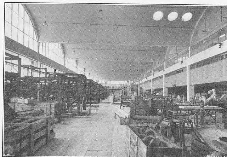
FIG. 4. MILL ROOM, LOOKING TOWARDS "BANBURY" CORNER.
