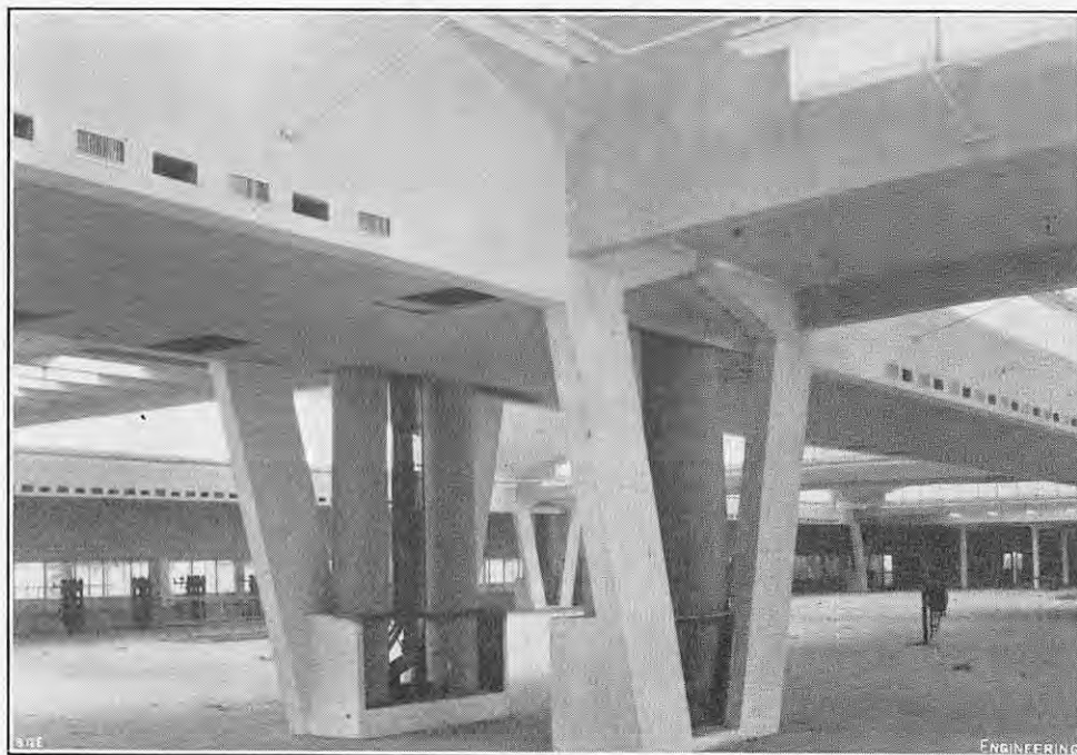
FIG. 9. PAIRS OF RAKING COLUMNS SUPPORTING ADJOINING DOMES.
