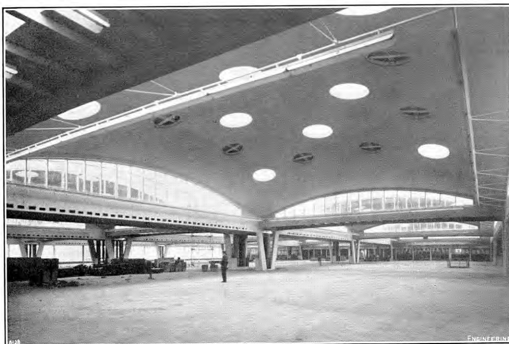
FIG. 6. DOMED ROOF OF MAIN PRODUCTION AREA.
