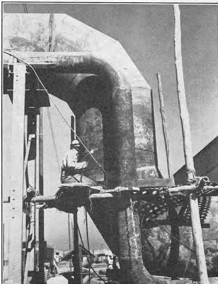
FIG. 10. OUTSIDE ERECTION AT SINDRI.
