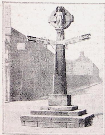
The conversion of the ancient cross at Crich, near Matlock, into a signpost is being severely criticised by local residents.
