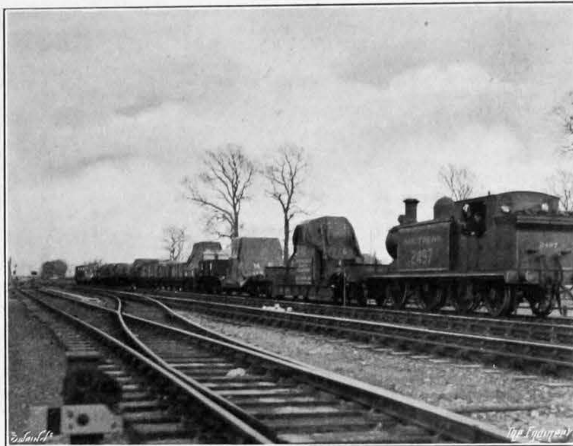
FIG. 6—SUB-STATION EQUIPMENT ON TRAIN
