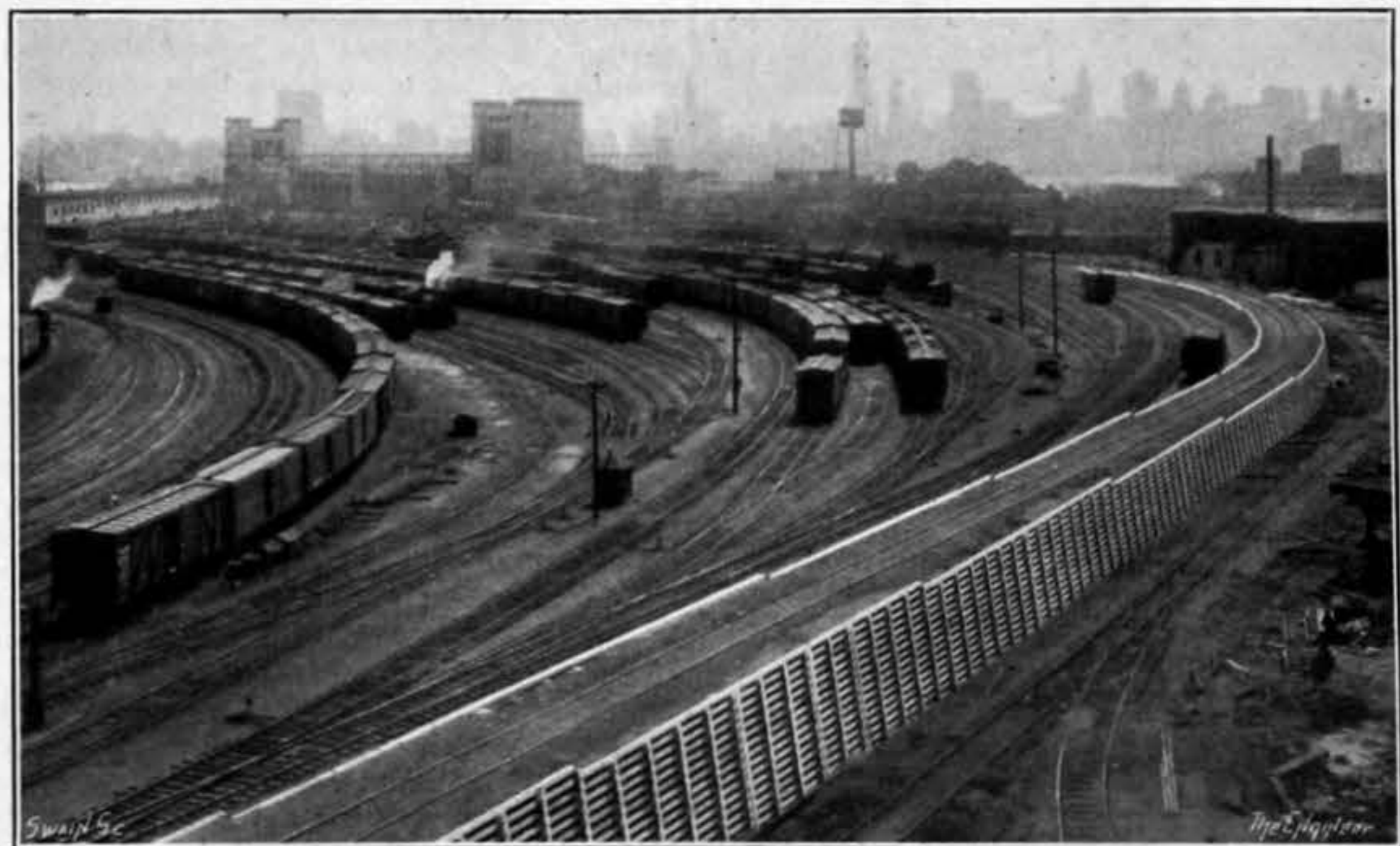
FIG. 1—CONCRETE CRIB WORK RETAINING WALL AT HOBOKEN
