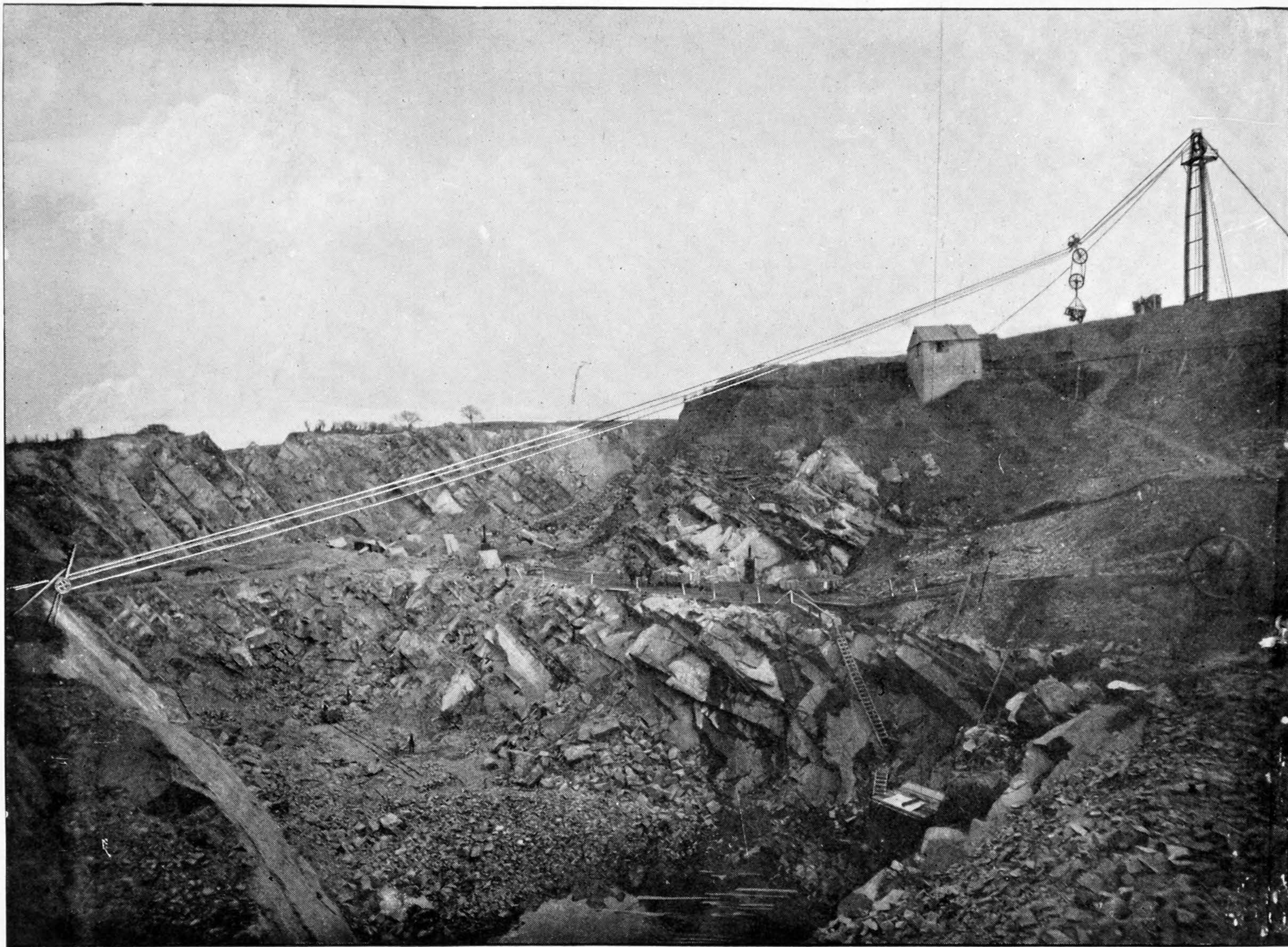
HENDERSON INCLINE CABLEWAY, STONEY STANTON, LEICESTERSHIRE. SPAN, 495 FT. ; LOAD, 3 TONS.
