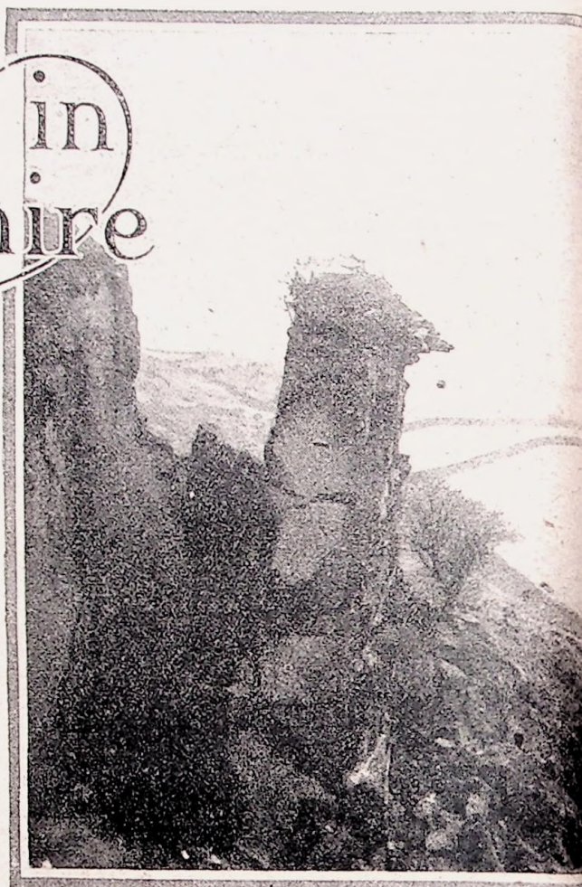
Hebden Falling Rock, which is steadily leaving the face of the cliff and may one day tumble down the hillside into the valley below.
