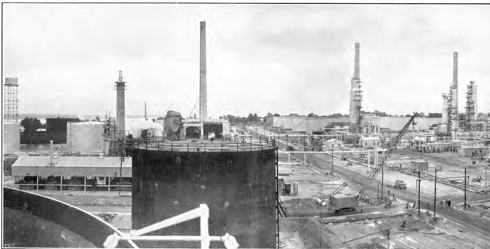
FIG. 8. GENERAL VIEW OF REFINERY AREA, SHOWING BOILER-HOUSE,
