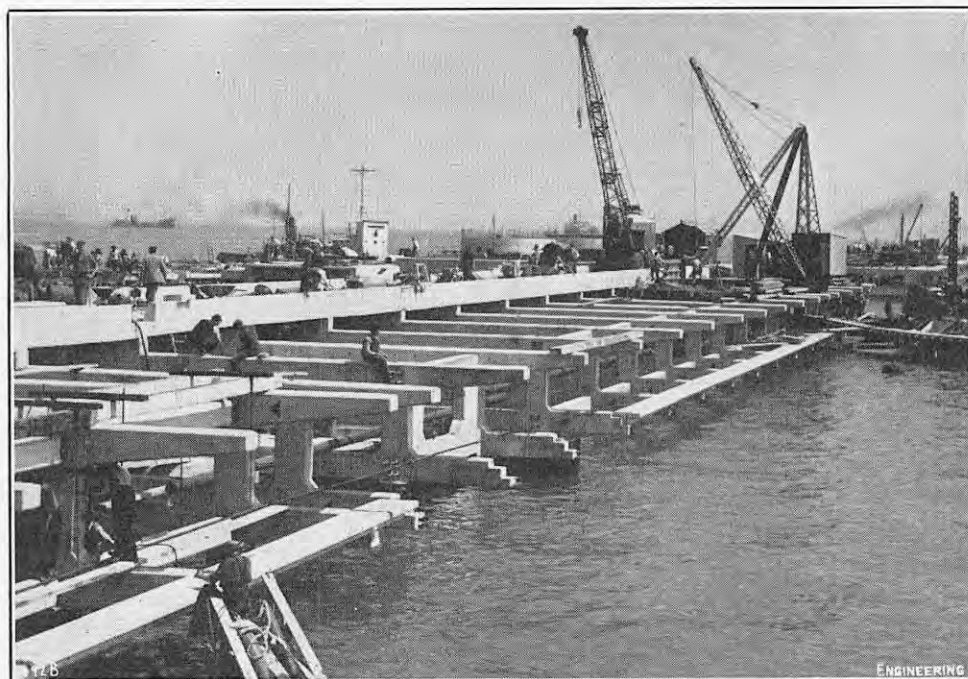
FIG. 2. JETTY UNDER CONSTRUCTION.
