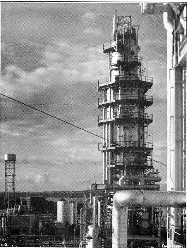
FIG. 11. SINGLE-STAGE FRACTIONATING COLUMN.
