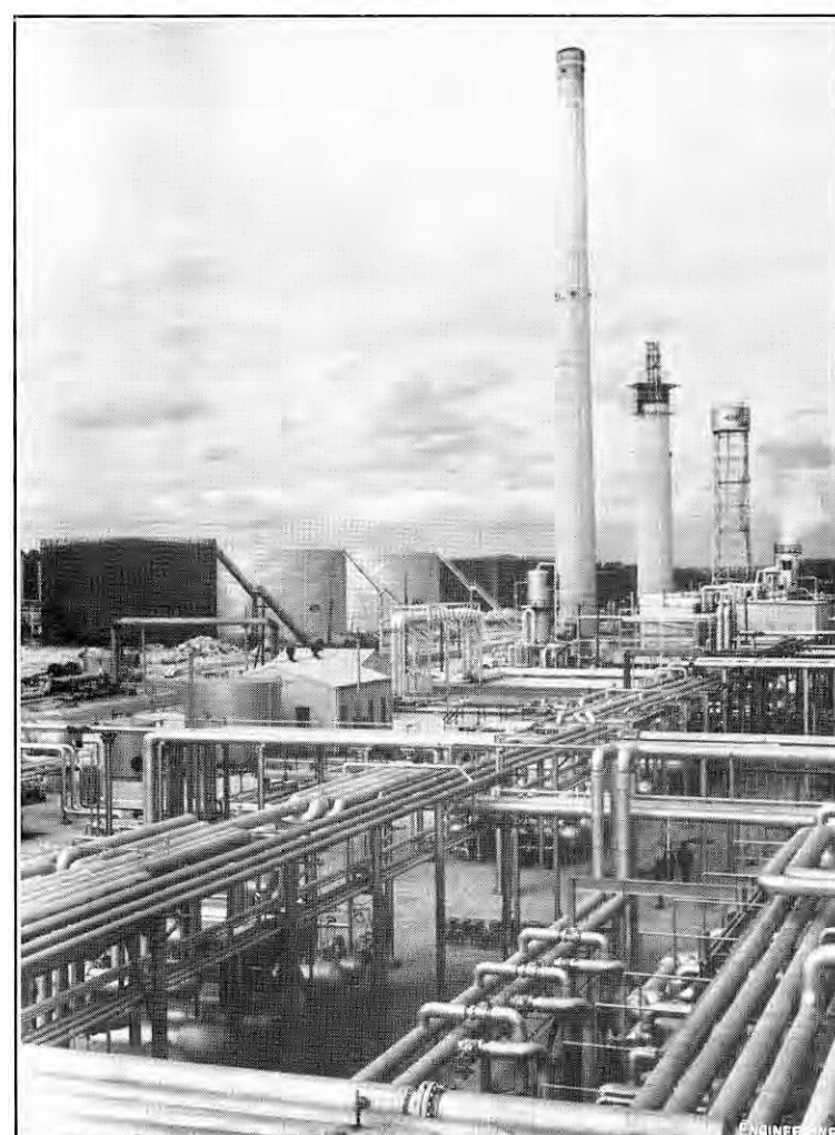
FIG. 16. PIPING FOR CRUDE-OIL UNITS.
