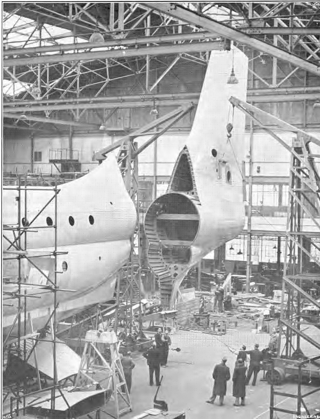
FIG. 11. ERECTING MAIN PART OF FIN ON HULL.
