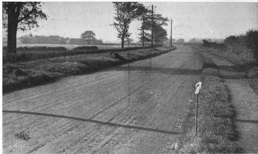
Another portion of the trapped York-Tadcaster Road taken from the York side. The distance over which cars are timed starts from the handkerchief in the foreground. These two views well illustrate what the police profess to regard as roads upon which a speed of over twenty miles an hour is "dangerous to the public."
