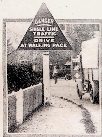
An arresting danger sign at the bottom of Dedham Gun hill, on the borders of Essex and Suffolk, where an old iron bridge is being rebuilt.
