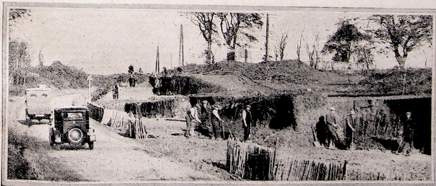
GREAT NORTH ROAD WIDENING.
