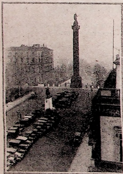
An aerial view of one of London's largest free car parks—Waterloo Place, with a most imposing statue towering high above it.
