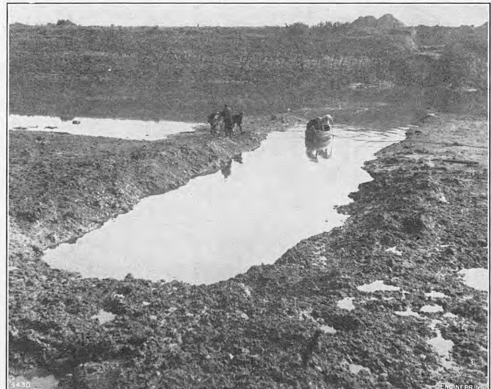
FIG. 4. SWANSEA END OF TRENCH.
