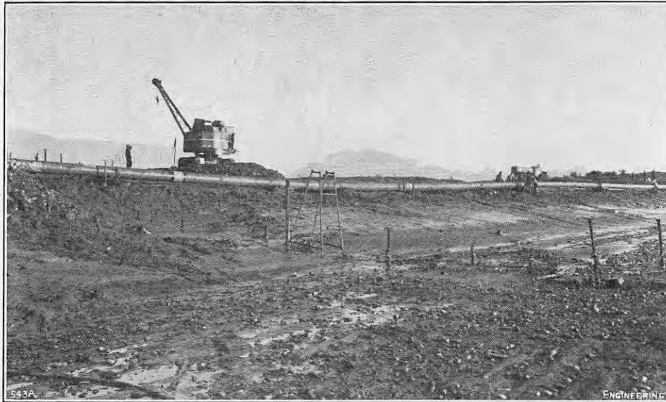
FIG. 1. PIPELINE ON RIVER BANK.
