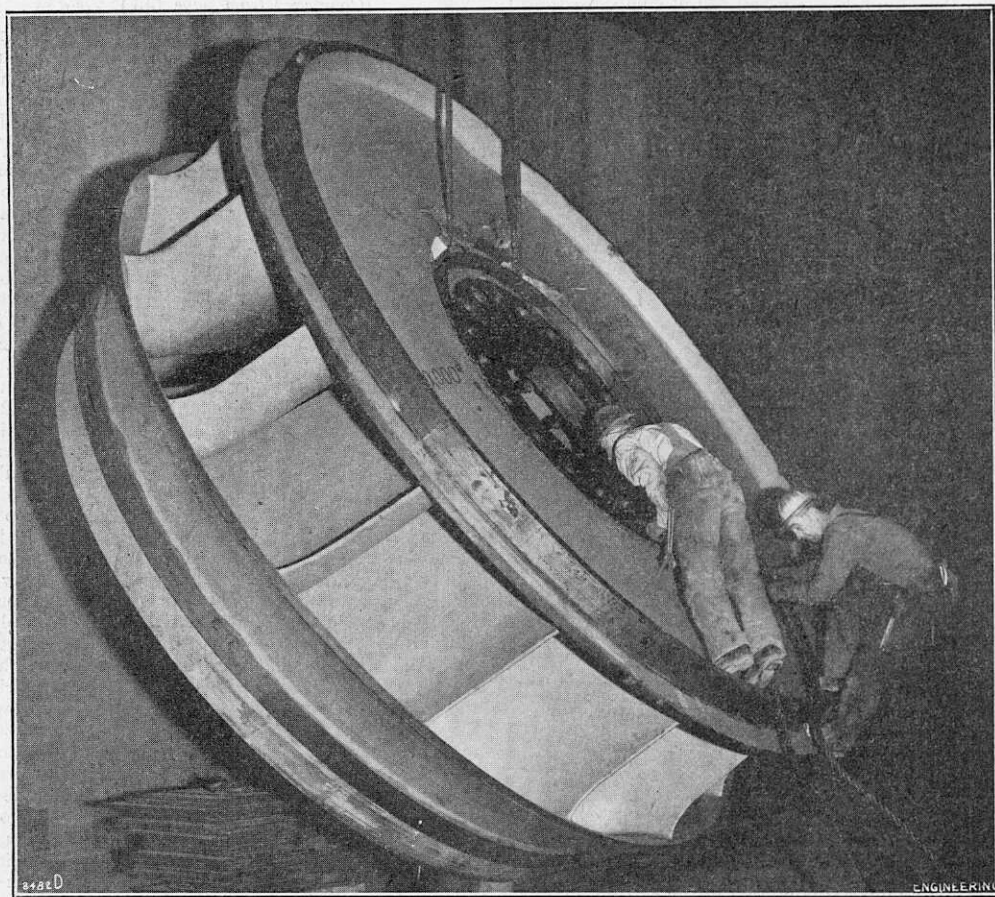
FIG. 17. TURBINE RUNNER.
