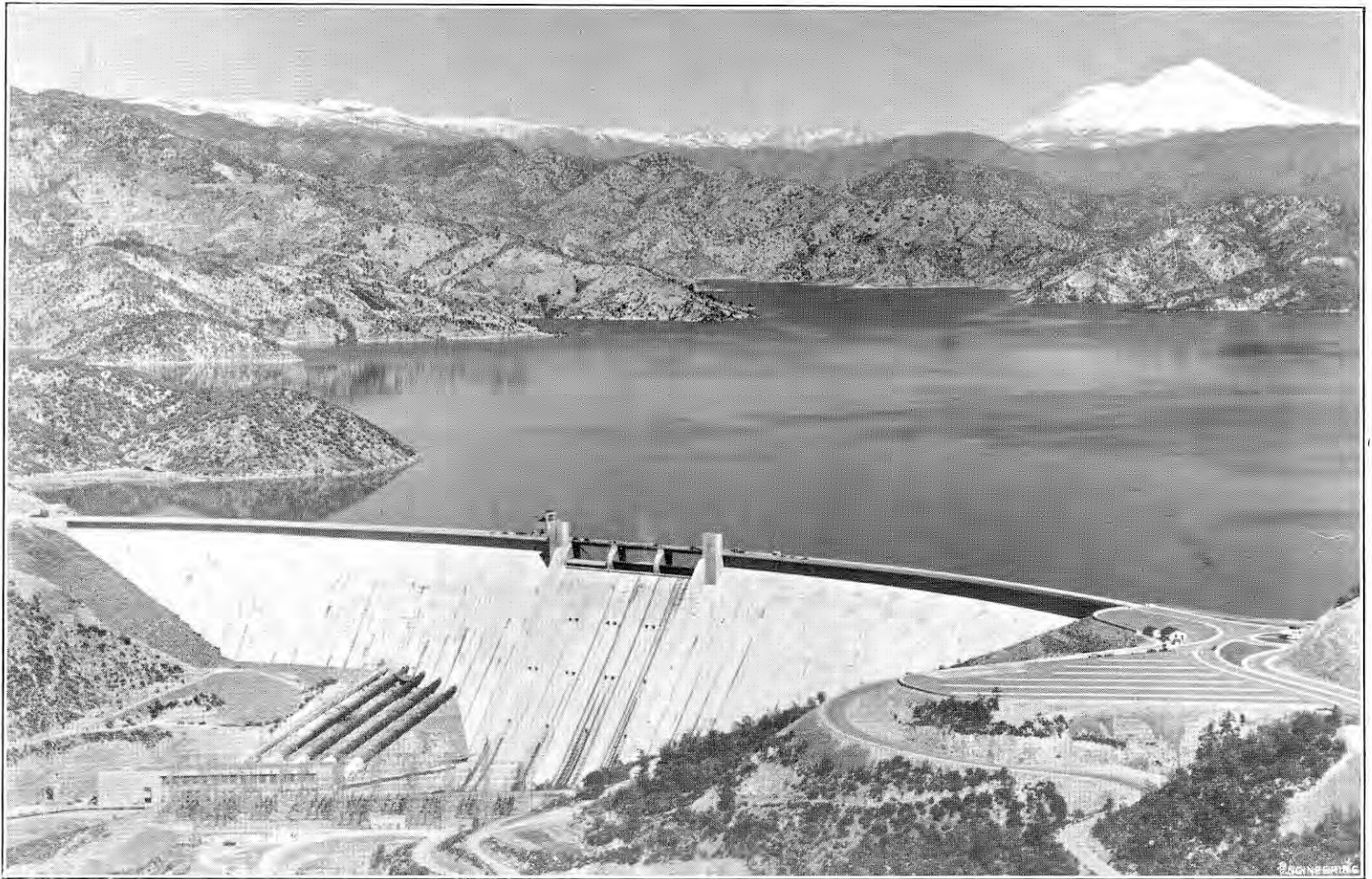
FIG. 2. SHASTA DAM AND LAKE, ON THE SACRAMENTO RIVER.
