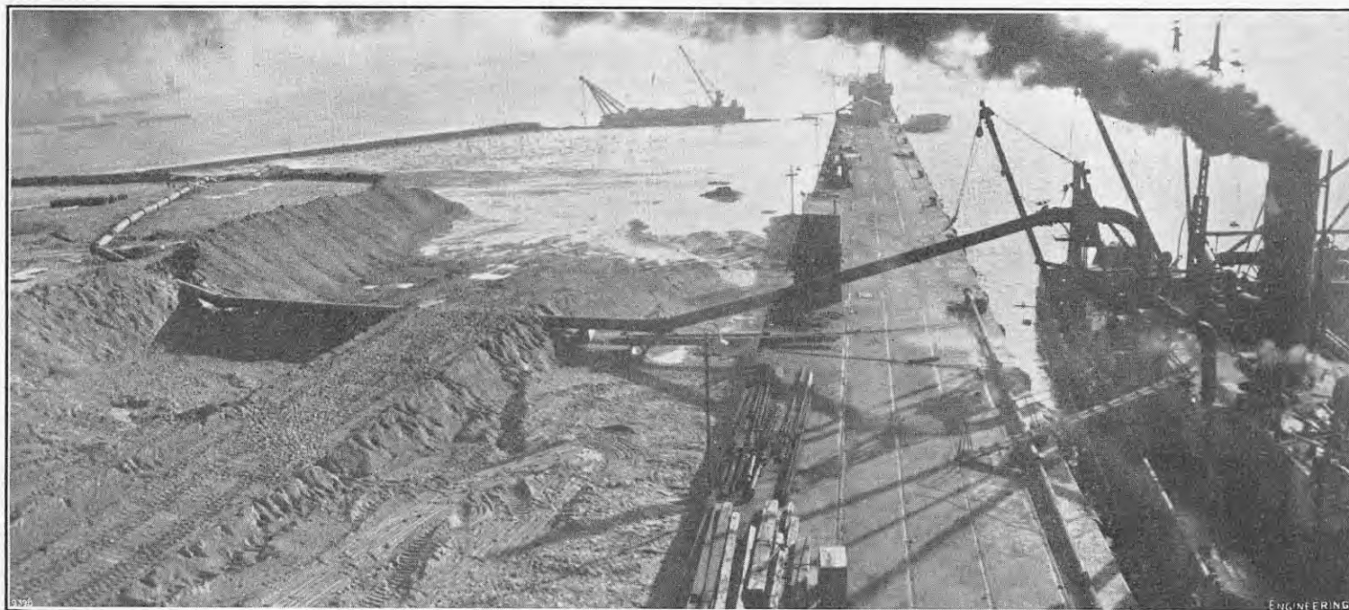
FIG. 2. RECLAMATION WORK BEHIND OCEAN PIER.
