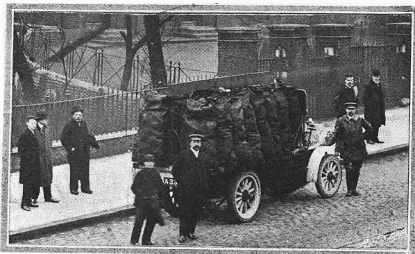
A single-cylinder engine Orion waggon on its way to the Agricultural Hall Show. The same waggon has during ten working days transported 104 tons of coal, distributing it around the suburbs of London.
