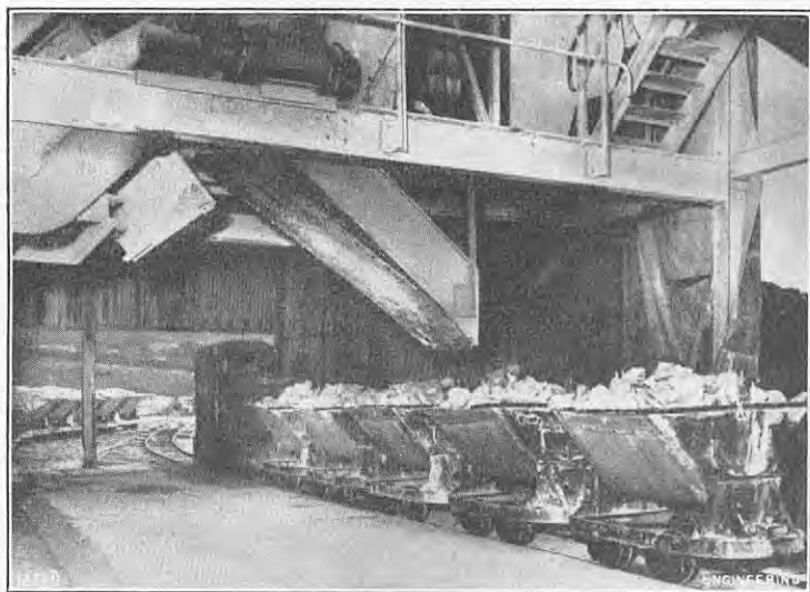
FIG. 4. LOADING CRUSHED AND SCREENED CHALK.
