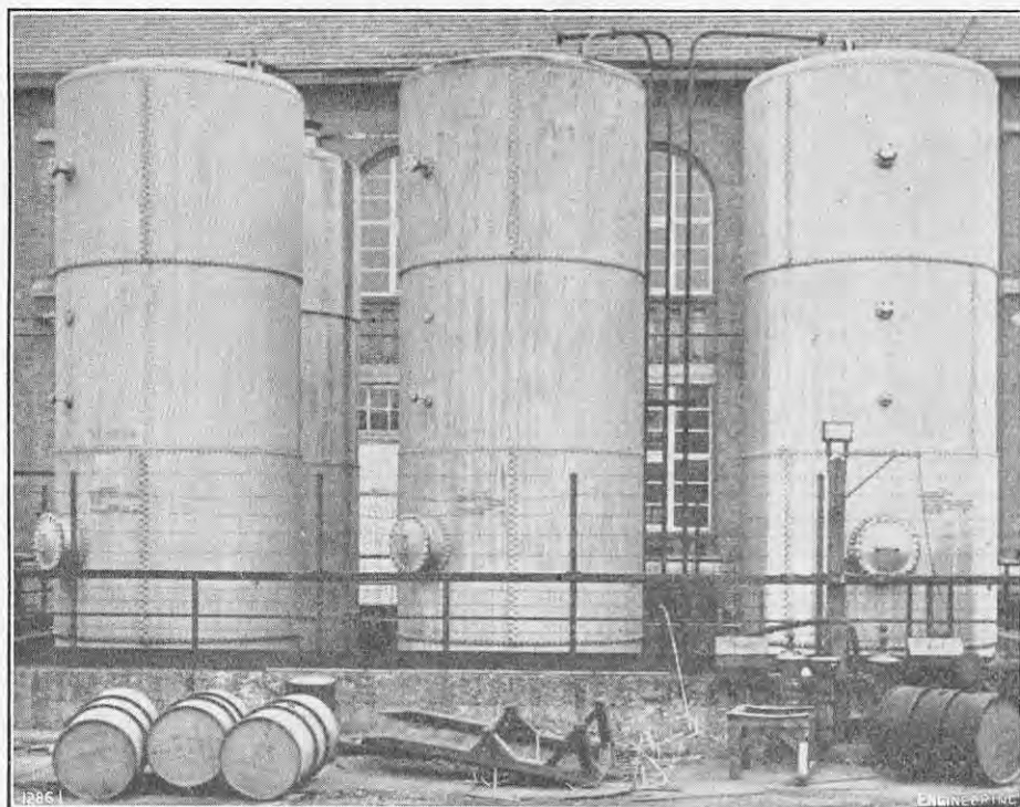
FIG. 9. TANKS TREATED WITH LEAD CYANAMIDE, AFTER 16 YEARS.
