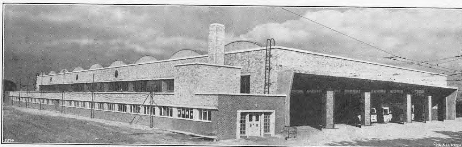
FIG. 1. GENERAL VIEW OF GARAGE.
