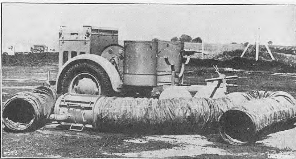
FIG. 2. FAN CONNECTED TO FLEXIBLE DUCTING.
