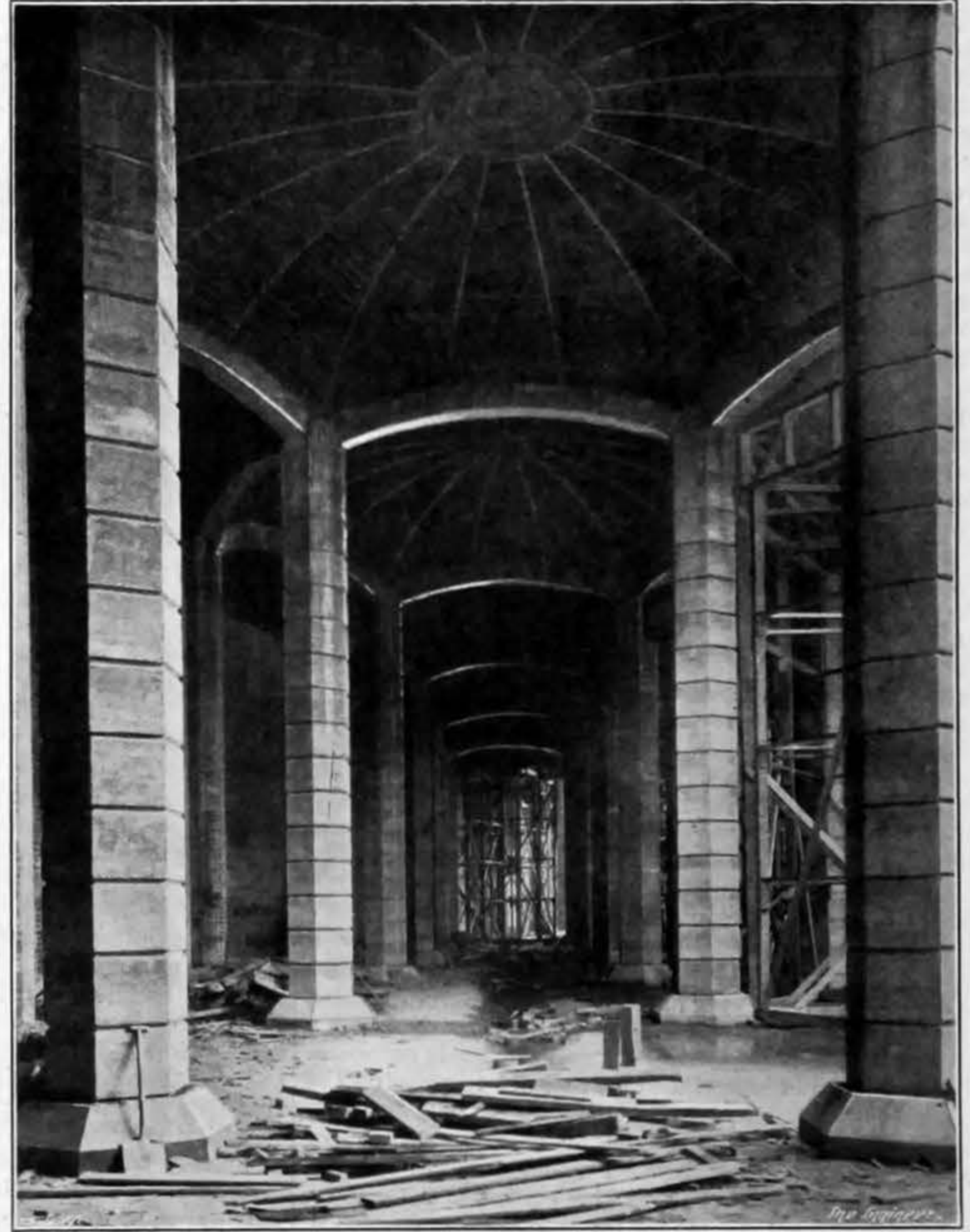
FIGS. 9 AND 10—INTERIOR VIEWS OF CROSS HILL RESERVOIR WITHOUT AND WITH ROOF
