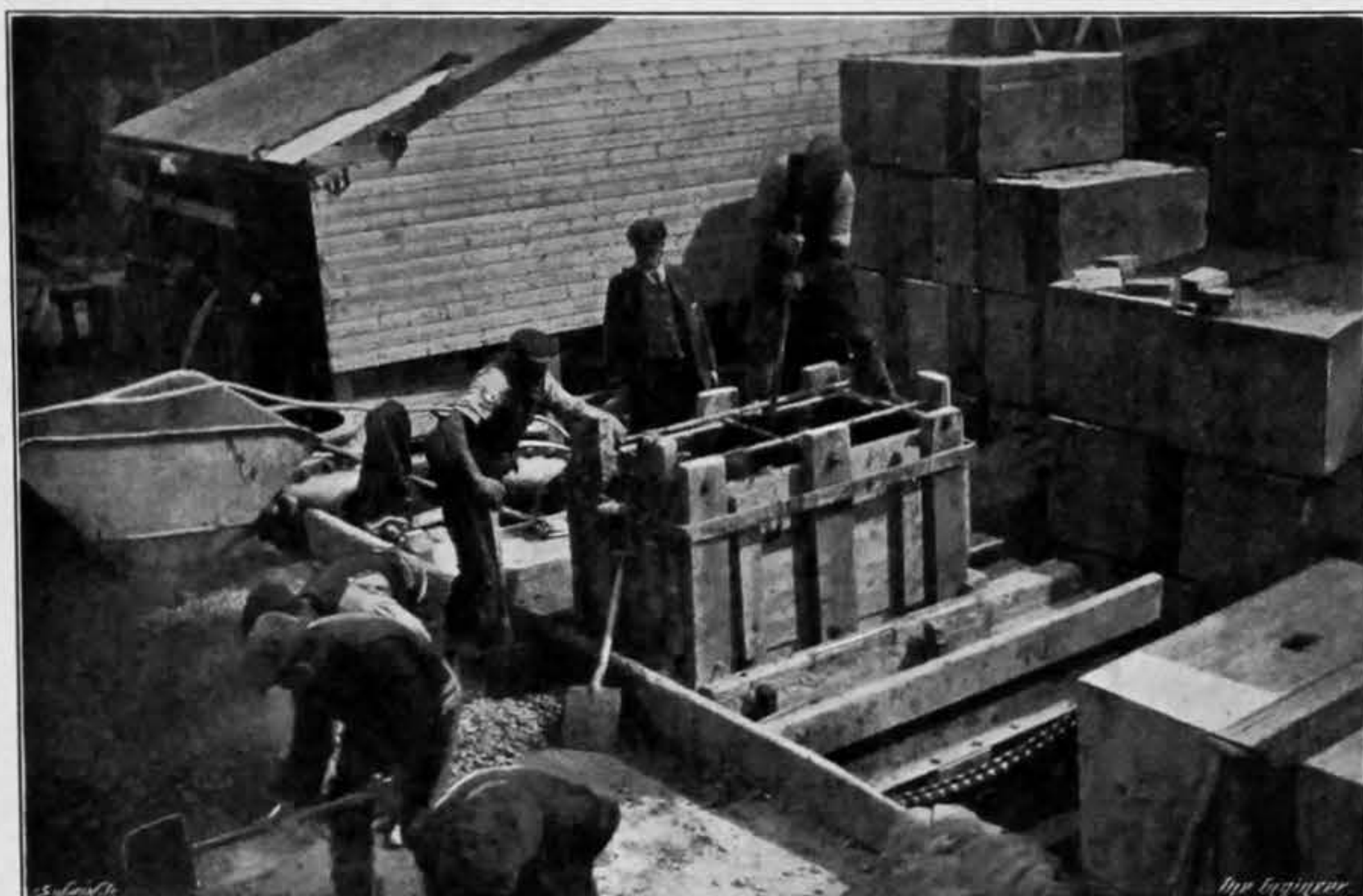
FIG. 5—BLOCK MOULD ON VIBRATING TABLE
