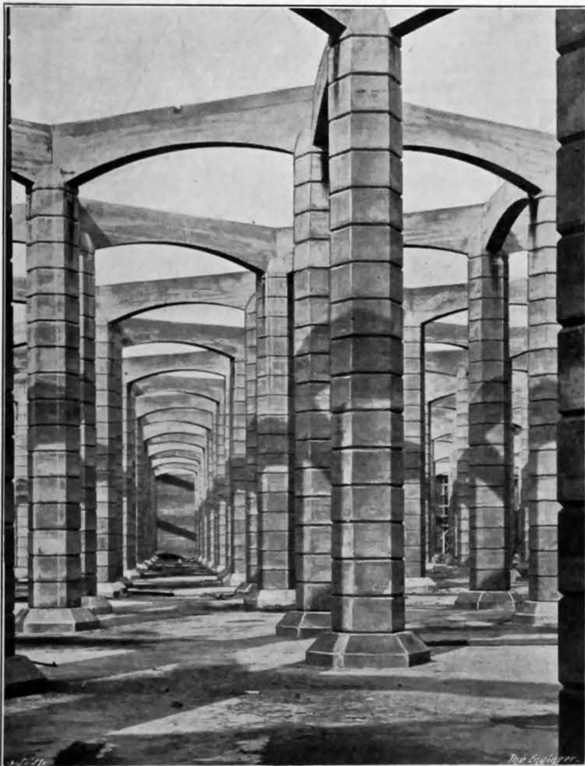
FIGS. 9 AND 10—INTERIOR VIEWS OF CROSS HILL RESERVOIR WITHOUT AND WITH ROOF
