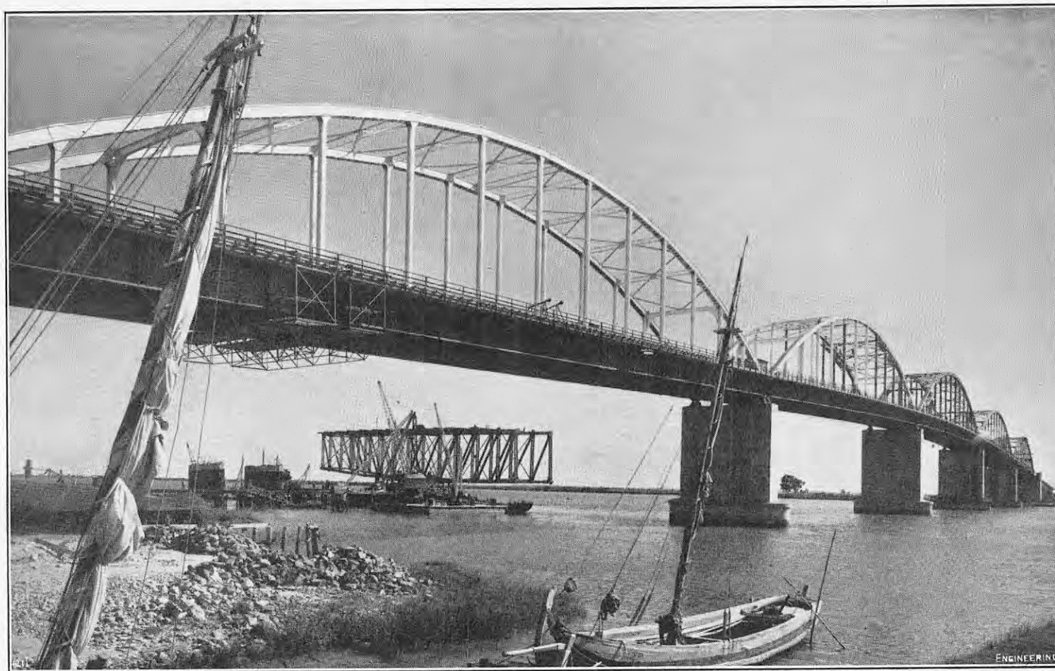
FIG. 35. ERECTION OF LAST SPAN COMPLETED.
