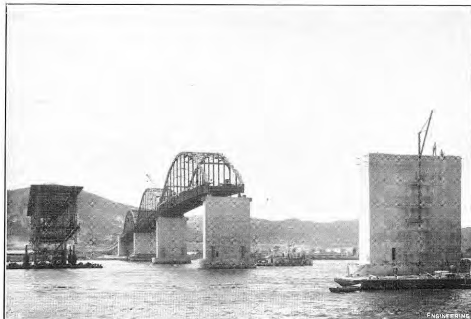
FIG. 31. SERVICE SPAN BEING REMOVED AFTER ERECTION OF SPAN "C."
