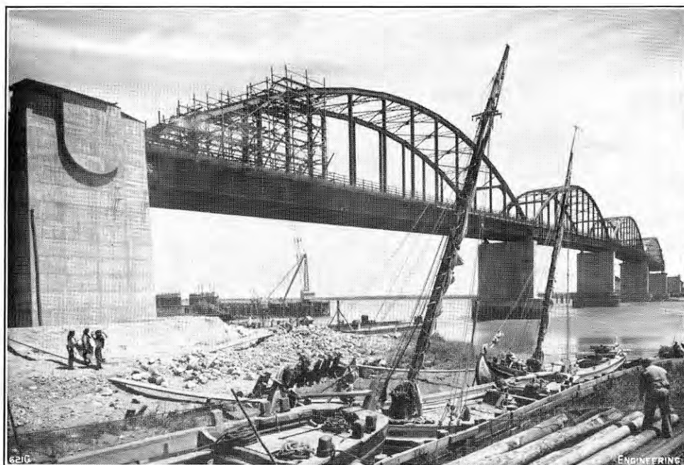
FIG. 33. VIEW OF BRIDGE FROM VILA FRANCA SIDE WITH FOUR SPANS ERECTED.
