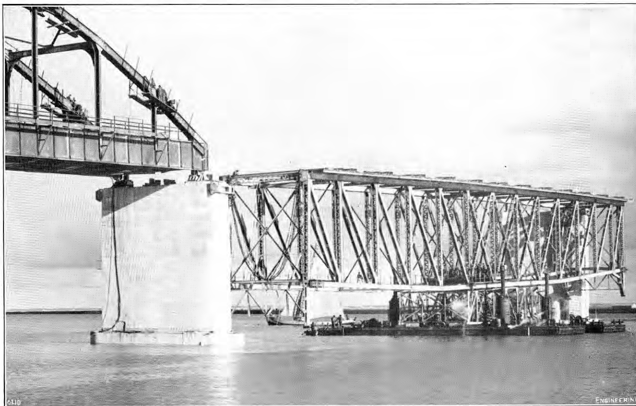
FIG. 30. SERVICE SPAN BEING MANEUVERED INTO POSITION FOR THE ERECTION OF SPAN "B."
