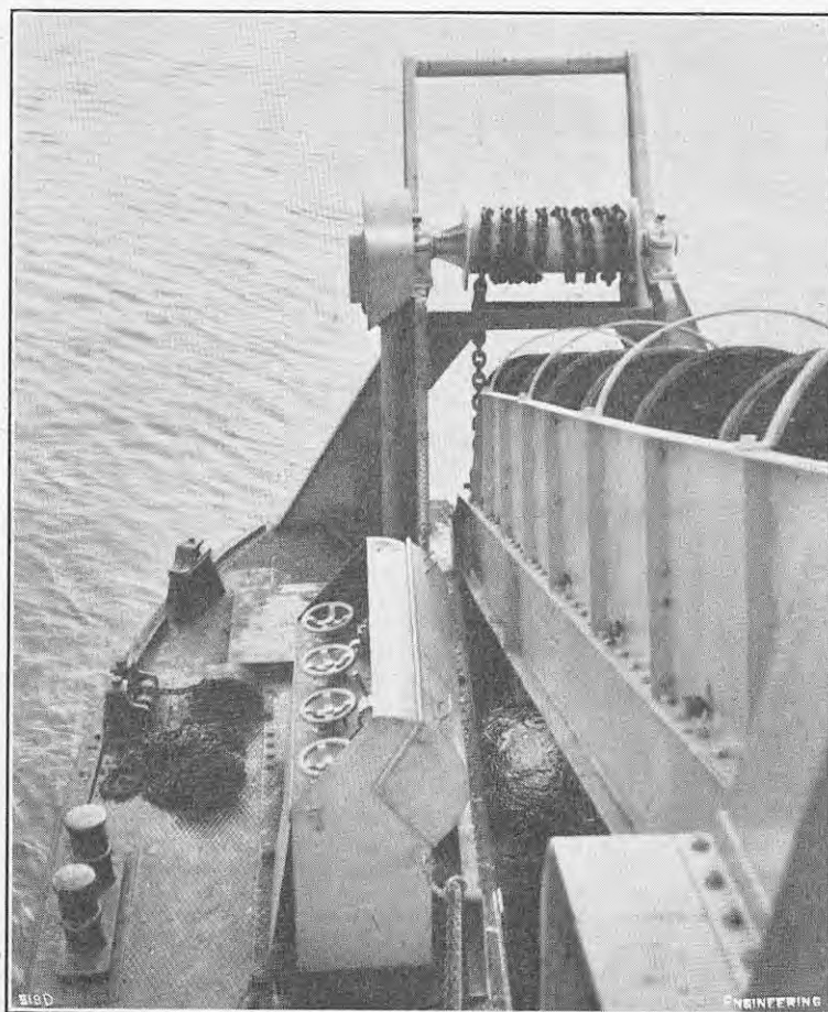
FIG. 6. WINCH CONTROL PANEL.
