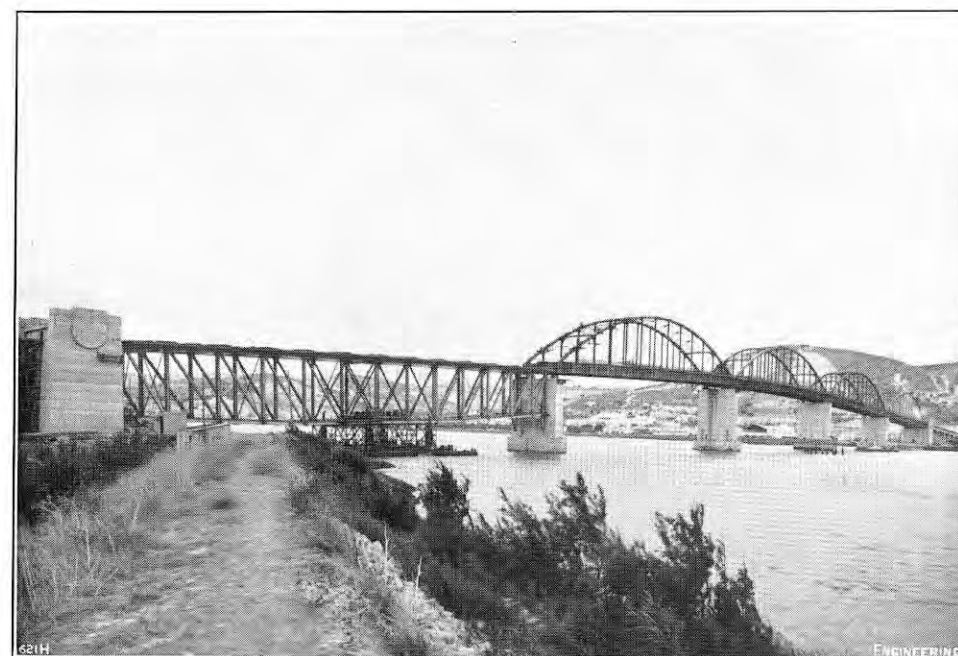
FIG. 34. SERVICE SPAN IN POSITION FOR ERECTION OF LAST ARCH SPAN.
