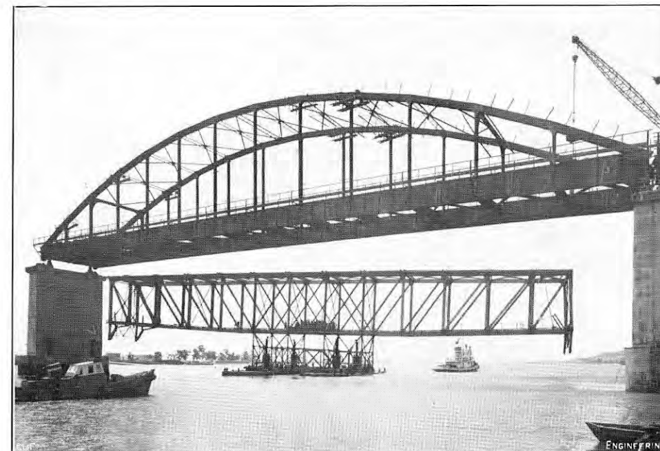
FIG. 32. SERVICE SPAN BEING MOVED FROM SPAN "C" TO SPAN "D."
