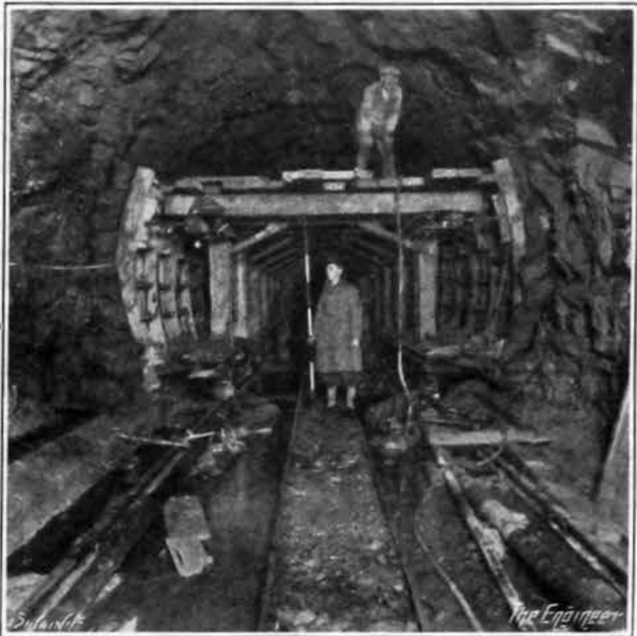
FIG. 31—CONCRETING CARRIAGE IN TUNNEL—MAY, 1933
