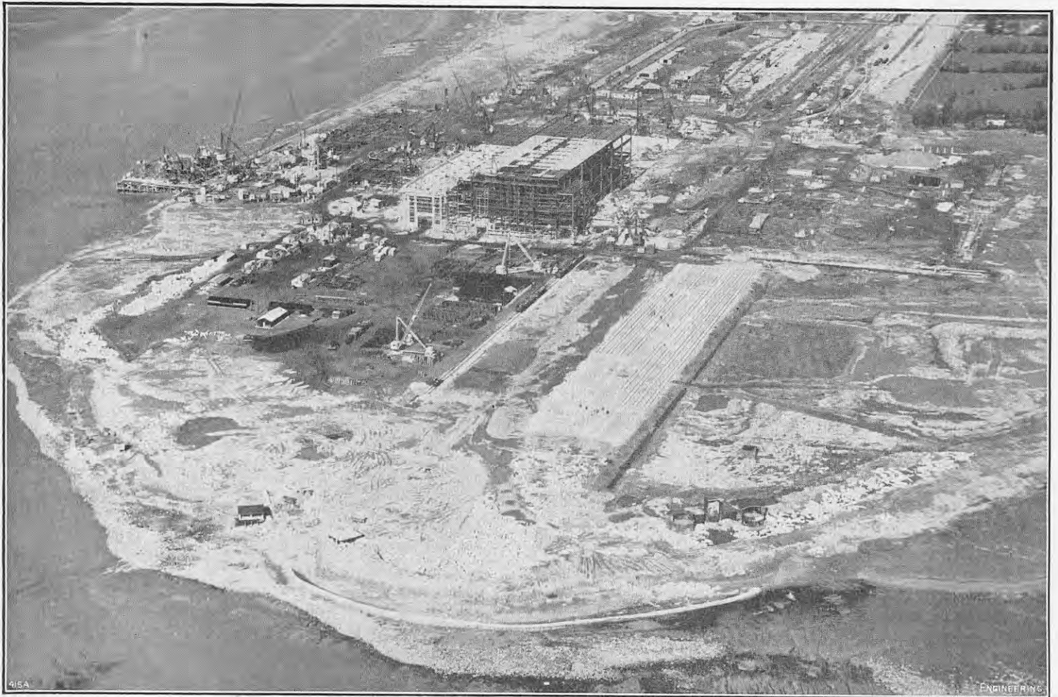
FIG. 1. AERIAL VIEW OF SITE.
