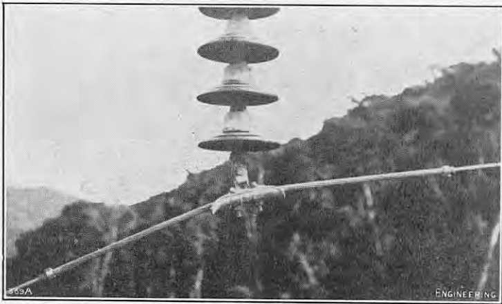
FIG. 1. PROTECTIVE COVERING OF CABLE.
