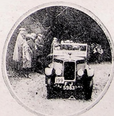
E. H. Williams (Triumph Super Seven) going well on Harcombe—one of the new hills.
