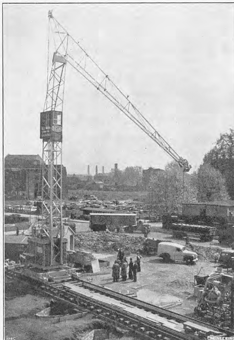
FIG. 3. RAISING JIB TO WORKING POSITION.
