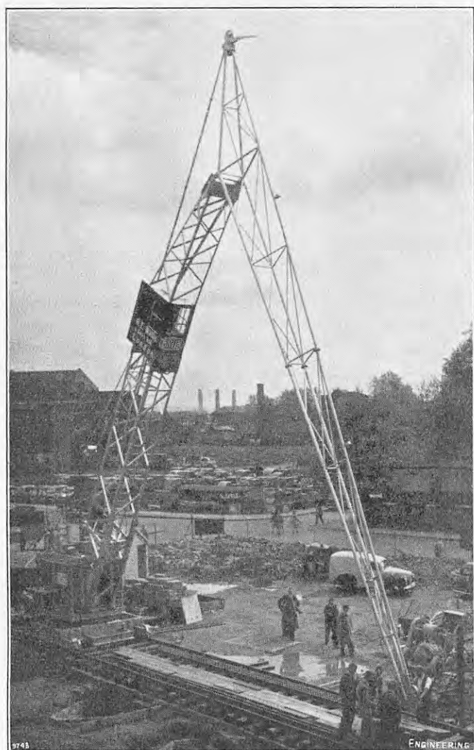
FIG. 2. HOISTING TOWER TO VERTICAL POSITION.
