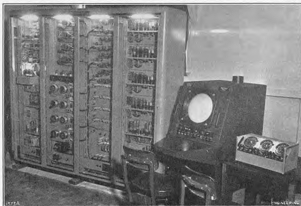
FIG. 1. CALCULATING EQUIPMENT AND REMOTE-CONTROL BOX.
