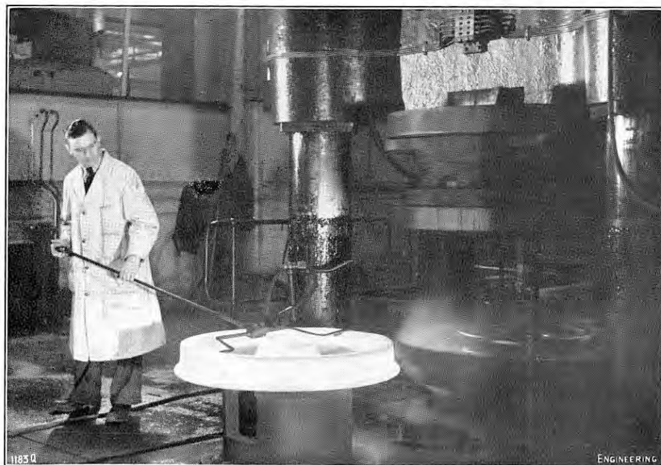
FIG. 20. GAUGING WHEEL AFTER DISHING.
