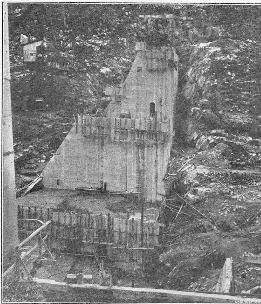
FIG. 19. BEINN A MHEADHOIN DAM UNDER CONSTRUCTION.
