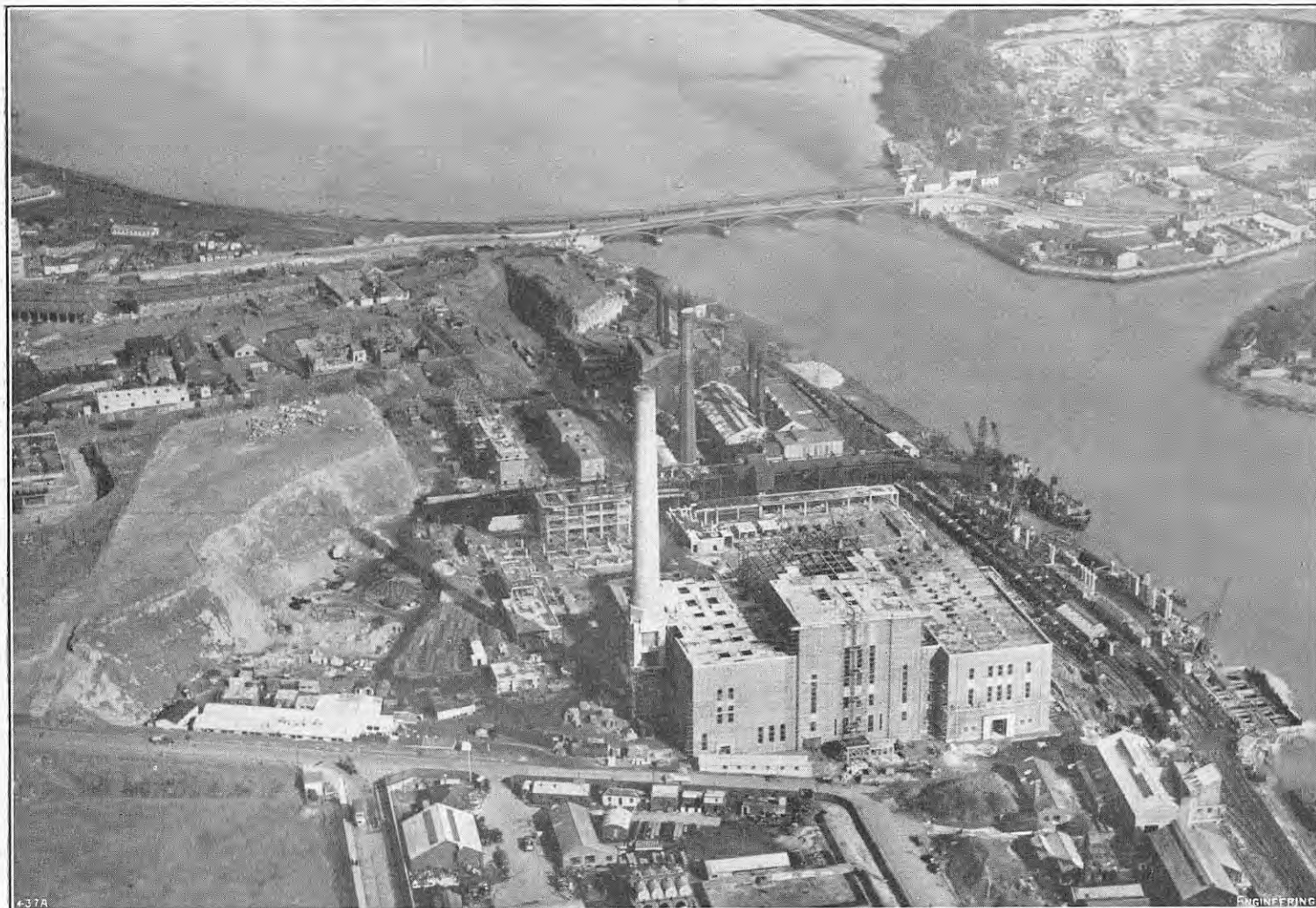
FIG. 1. GENERAL VIEW OF STATION AND SITE.
