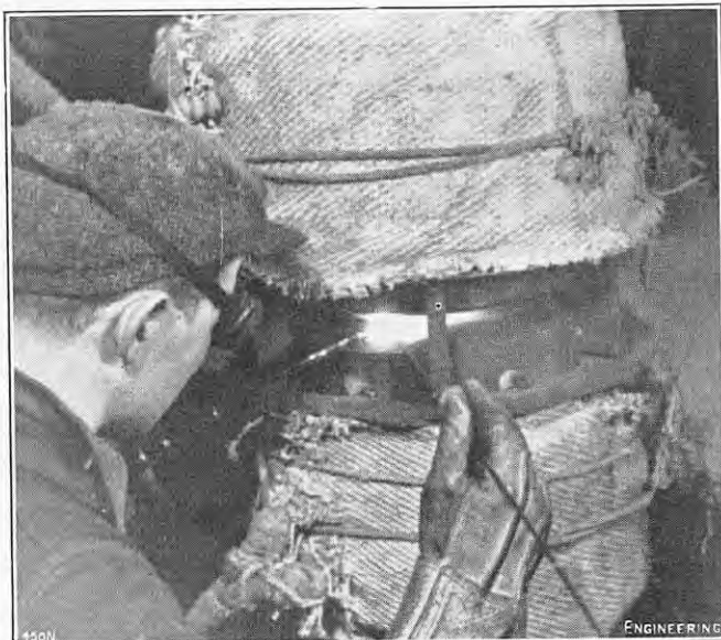
FIG. 13. ELECTRICAL-RESISTANCE PREHEATERS FOR WELDS.
