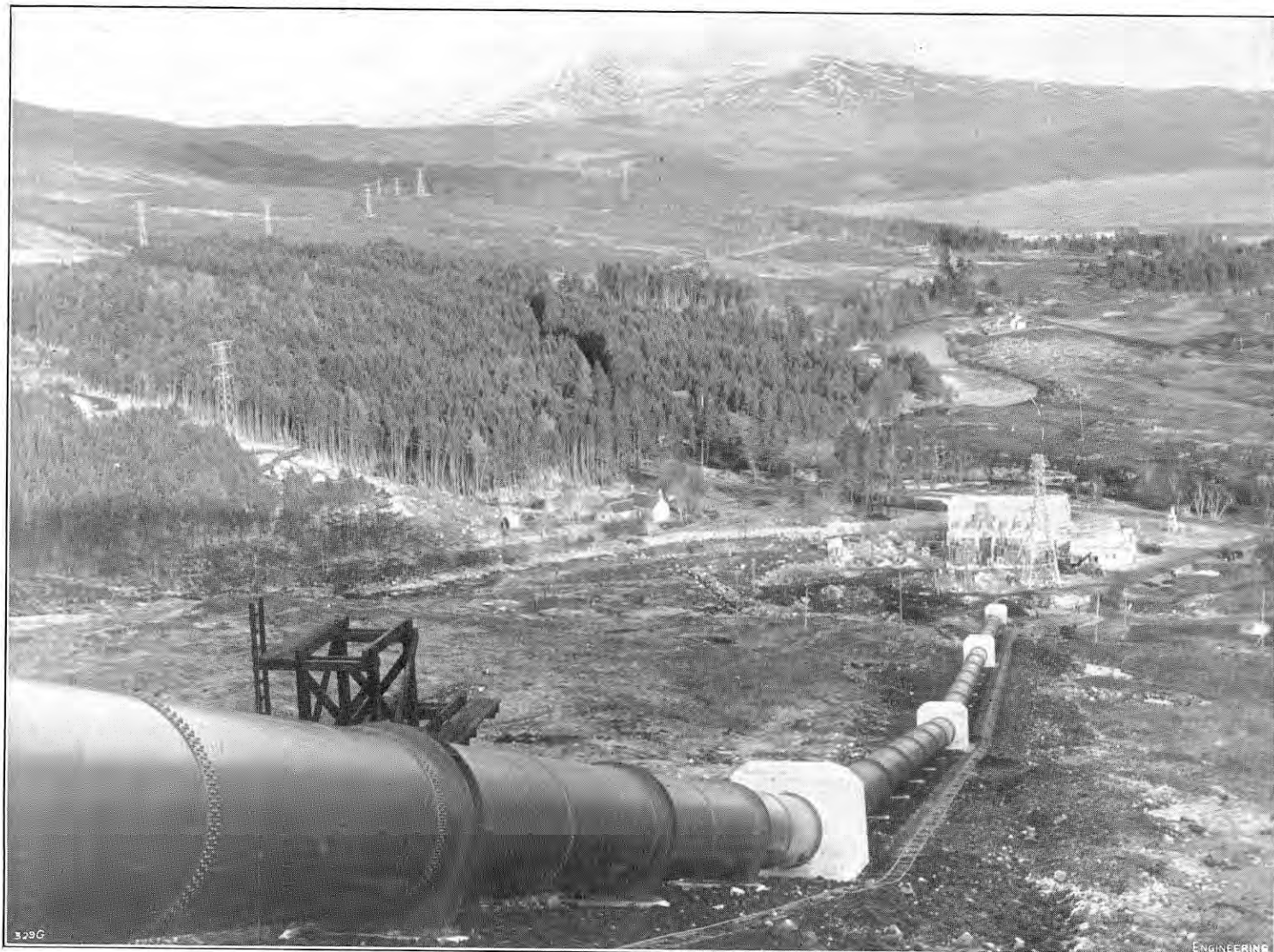
FIG. 29. PIPE LINE AND GRUDIE BRIDGE POWER STATION.
