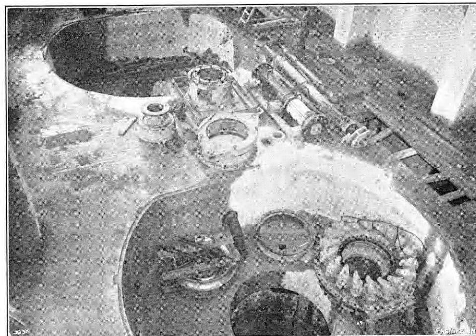
FIG. 32. TURBINE IN COURSE OF ERECTION.
