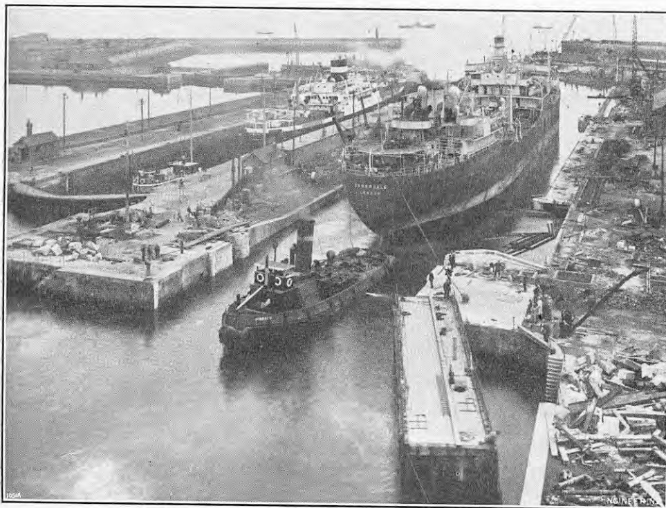
FIG. 1. PARTLY-RECONSTRUCTED DOCK IN USE.
