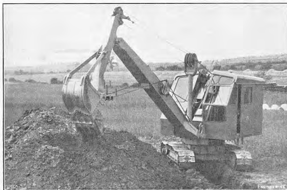
FIG. 21. EXCAVATOR WITH TRENCHING BUCKET ; PRIESTMAN BROTHERS, LTD.
