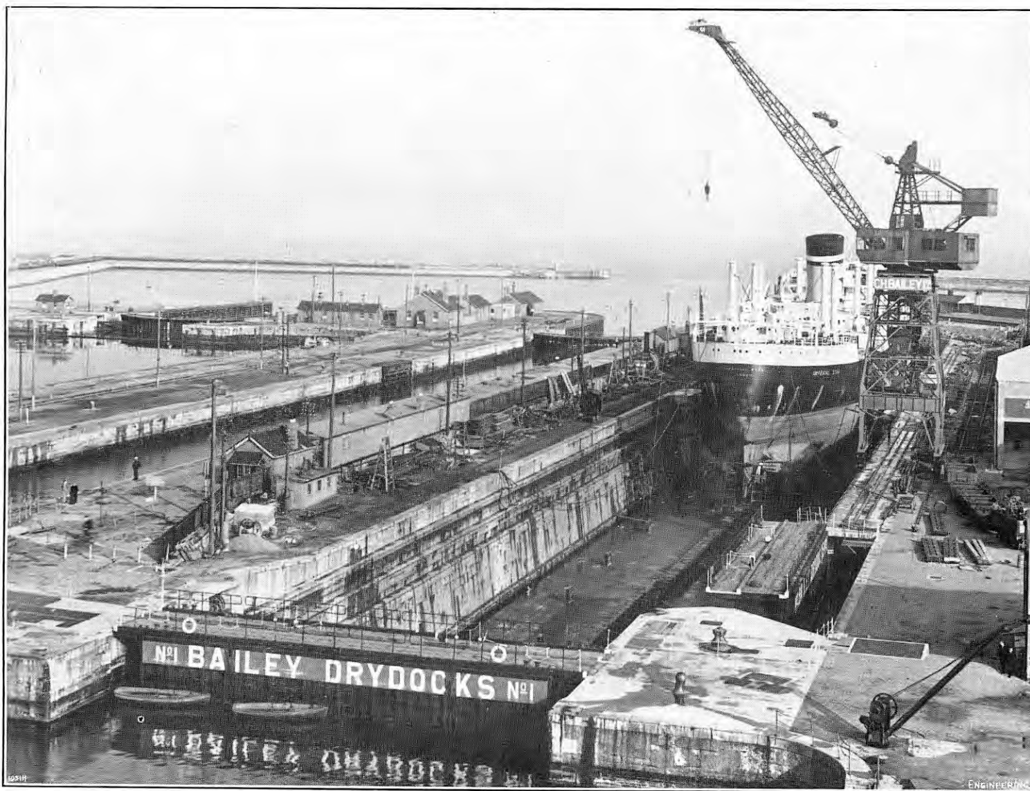
FIG. 8. DOCK IN USE.
