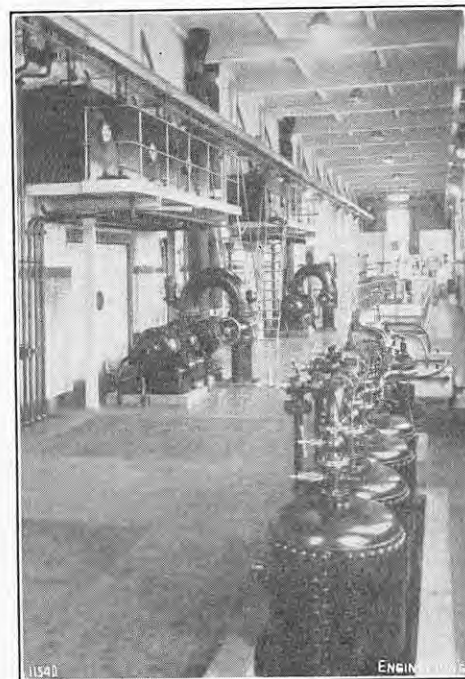
FIG. 4. SUPERCHARGERS AND COMPRESSED-AIR RECEIVERS.
