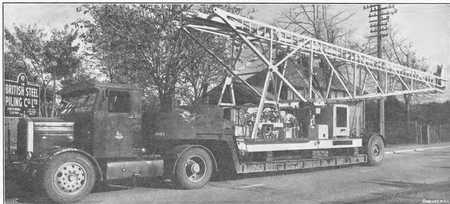
FIG. 20. PORTABLE PILE DRIVER ; BRITISH STEEL PILING CO., LTD.
