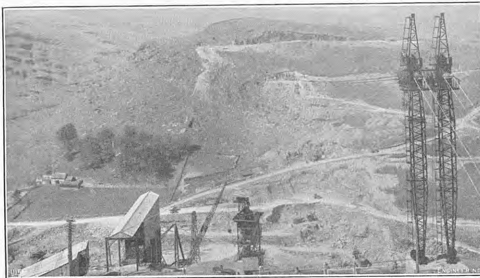
FIG. 4. SITE AT THE COMMENCEMENT OF THE WORK.
