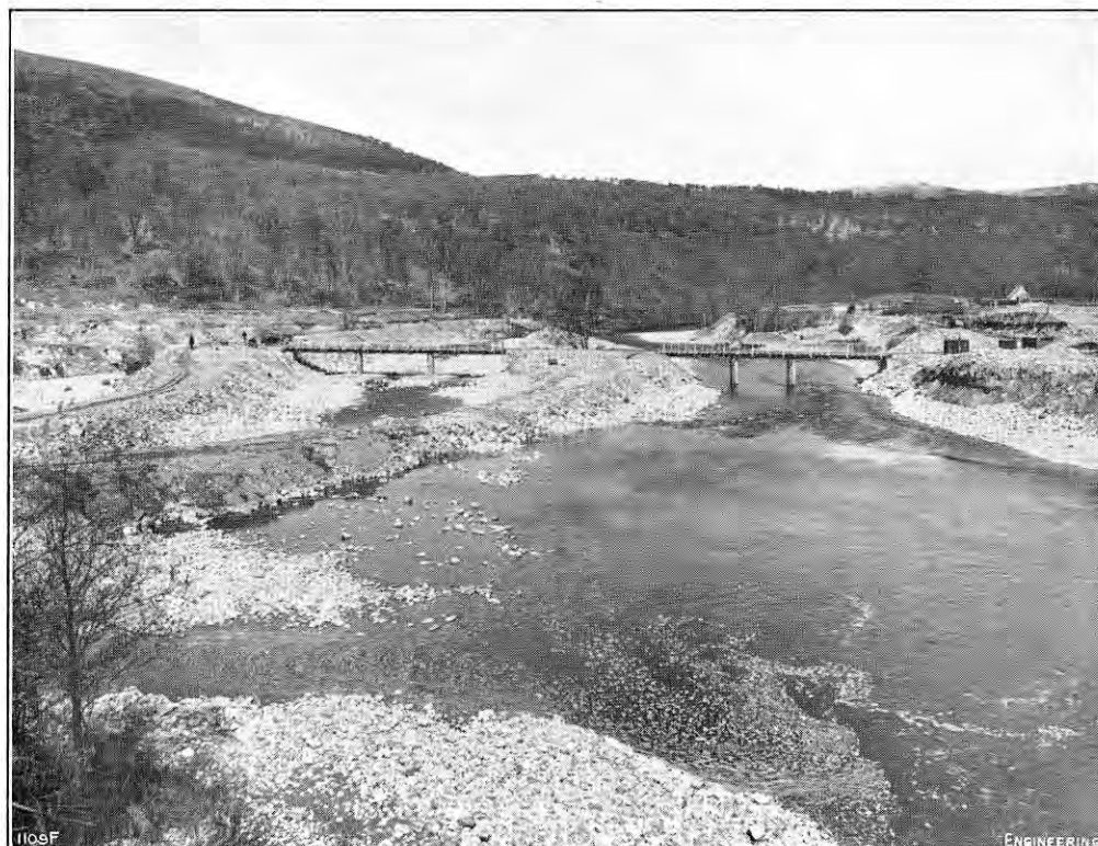
FIG. 42. DOWNSTREAM VIEW OF RIVER DIVERSION.
