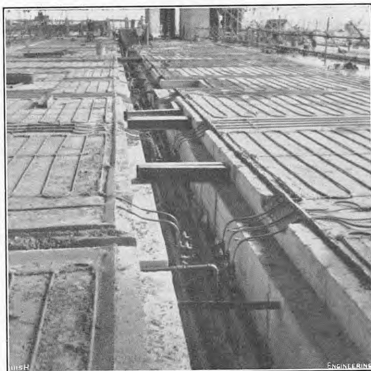
FIG. 10. HANGAR FLOOR HEATING COILS.
