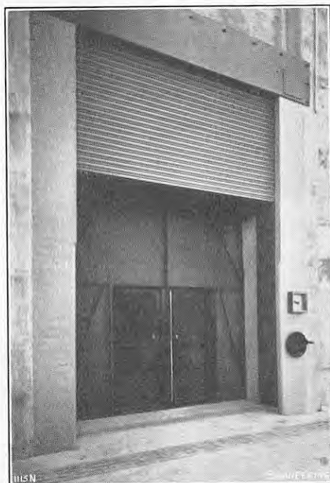
FIG. 11. HANGAR ACCESS DOOR, SHOWING FIREPROOF SHUTTER.
