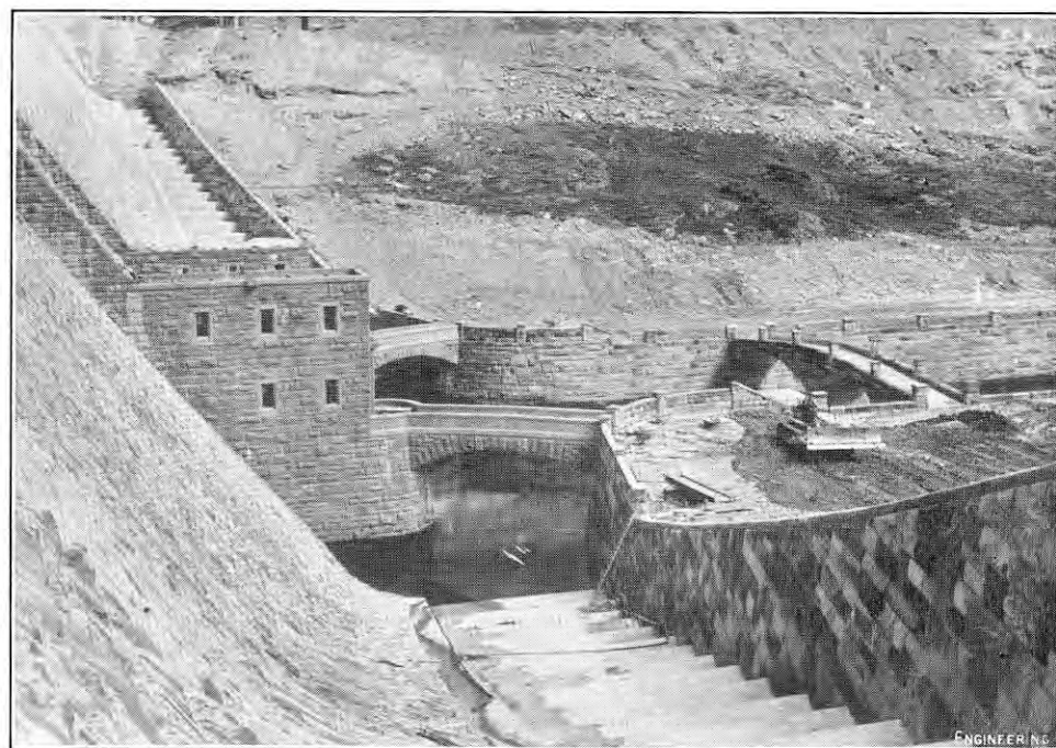
FIG. 12. VALVE HOUSE AT FOOT OF SPILLWAY.
