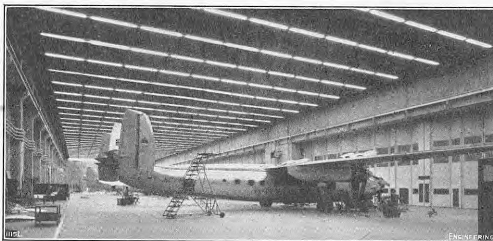
FIG. 14. HANGAR ILLUMINATED BY COLD-CATHODE LIGHTING.
