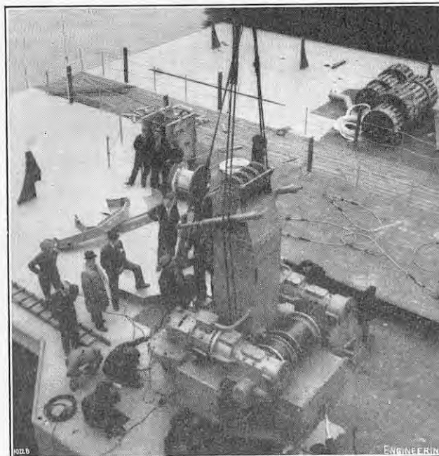
FIG. 2. ERECTION OF 3-TON CRANE.
