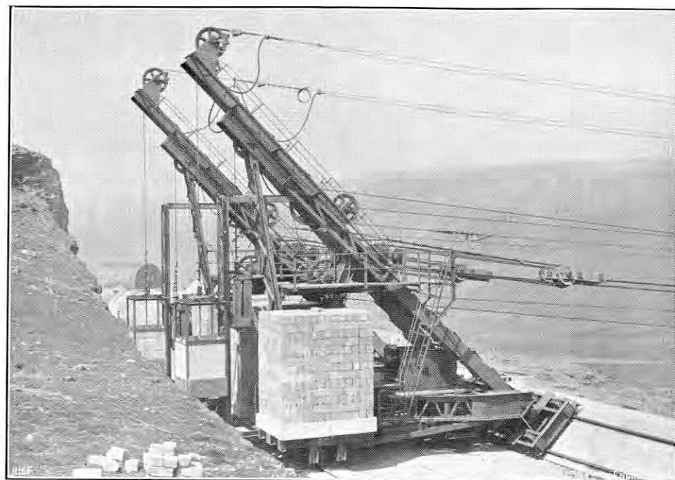
FIG. 10. TAILPOSTS OF CABLEWAYS.
