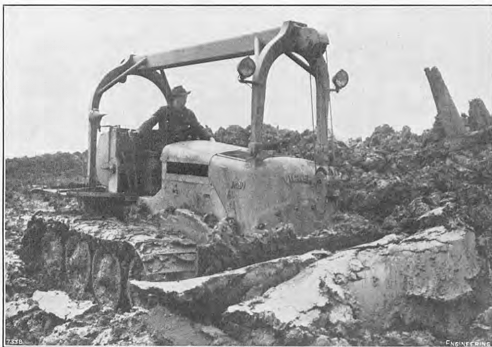
FIG. 2. TRACTOR AT WORK WITH BULLDOZING ATTACHMENT.
