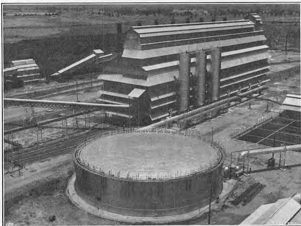
FIG. 1. SEMI-WATER-GAS PLANT AND GASHOLDER.
