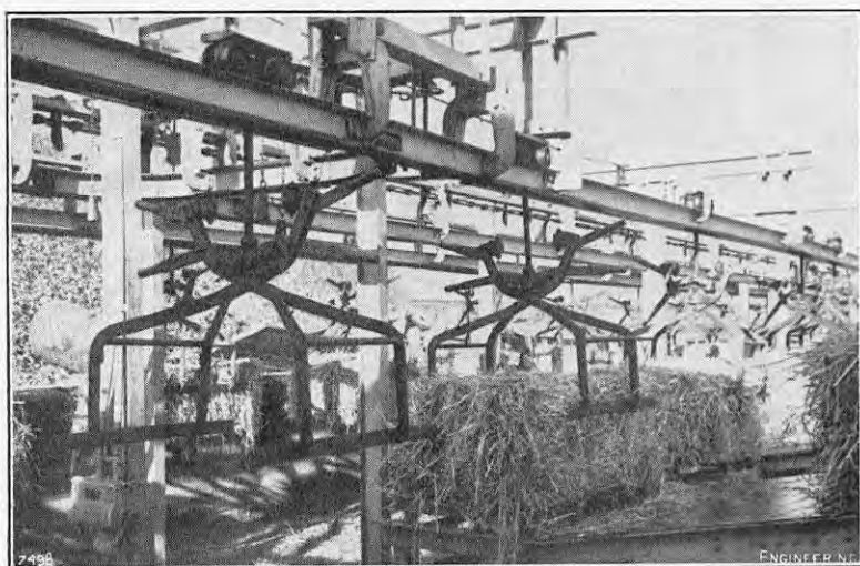
FIG. 2. LOADING BALES ON TO CONVEYOR.
