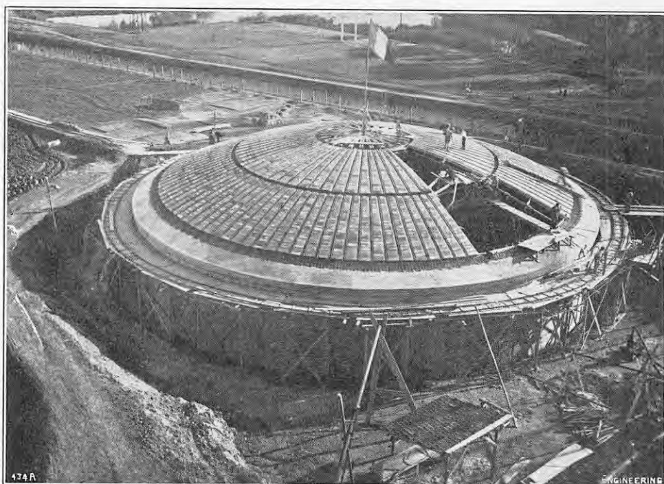
FIG. 1. CASTELLI TYPE OF OIL TANK.
