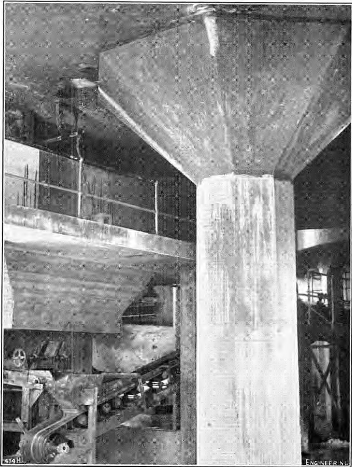
FIG. 9. HOPPER BELOW ROUGH MILLS.
