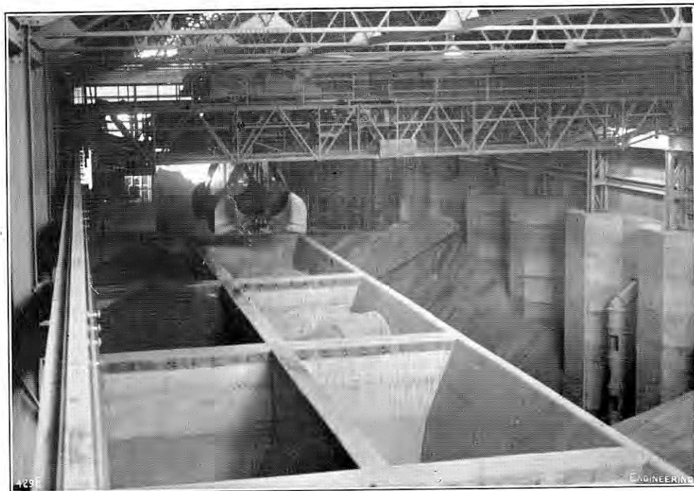
FIG. 17. INTERIOR OF STORE BUILDING.
