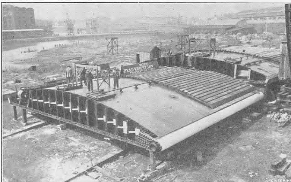
FIG. 1. DOCK GATE UNDER CONSTRUCTION.
