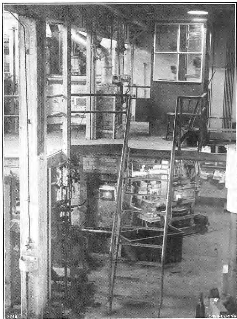
FIG. 2. GENERAL VIEW OF INSTALLATION.
