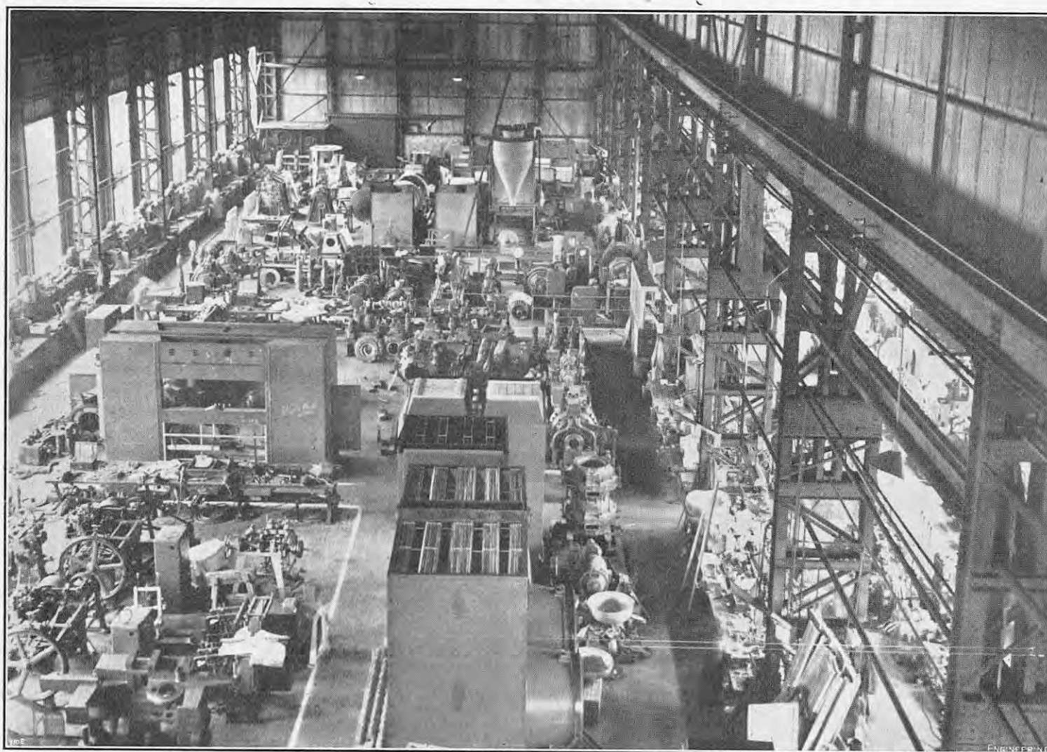
FIG. 5. LIGHT FITTING SHOP, WITH WATER-COOLERS IN COURSE OF ERECTION.
