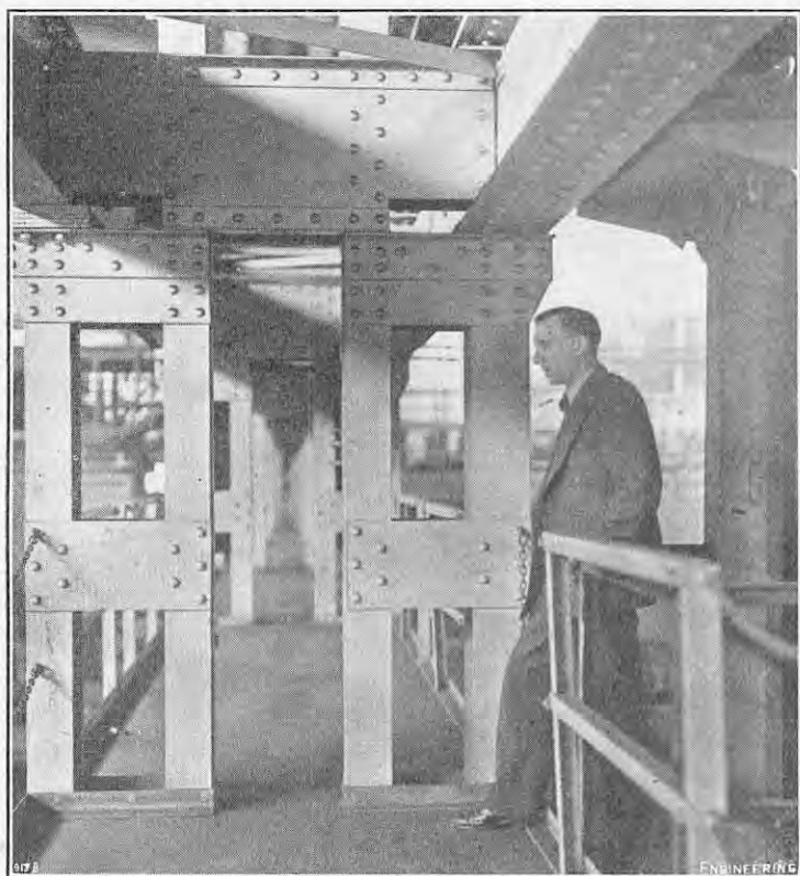
FIG. 11. WALKWAY FOR ACCESS TO CRANES.
