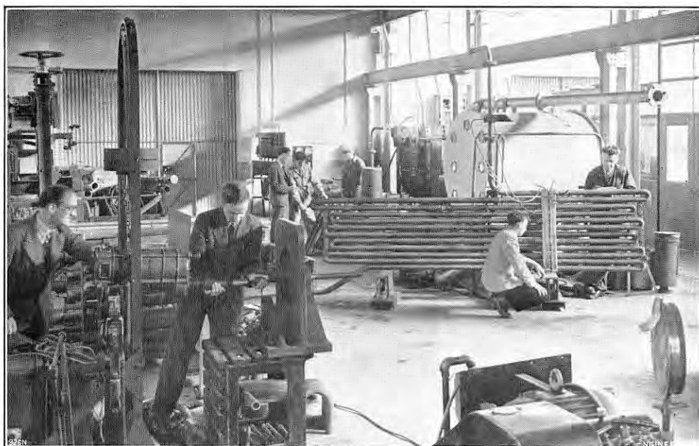
FIG. 16. ENGINEERING RESEARCH BAY.
