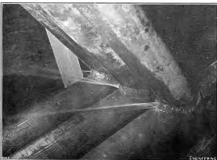
FIG. 21. WELDS TESTED TO FAILURE BY CYCLIC STRESS REVERSAL.
