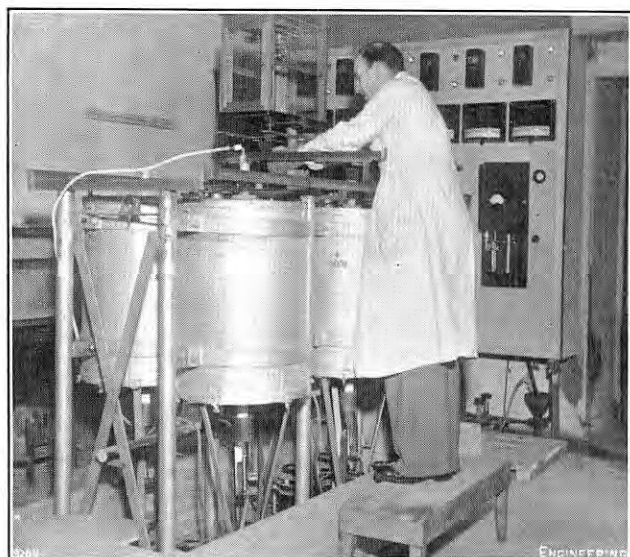
FIG. 23. TESTING FOR HIGH-TEMPERATURE SCALE.
