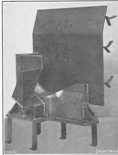
FIG. 12. BEARING SHOE FOR DOCK GATE.
