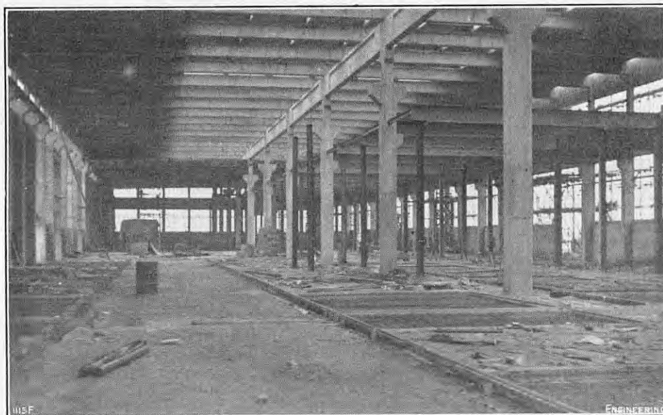
FIG. 7. THE WEST ANNEXE UNDER CONSTRUCTION.
