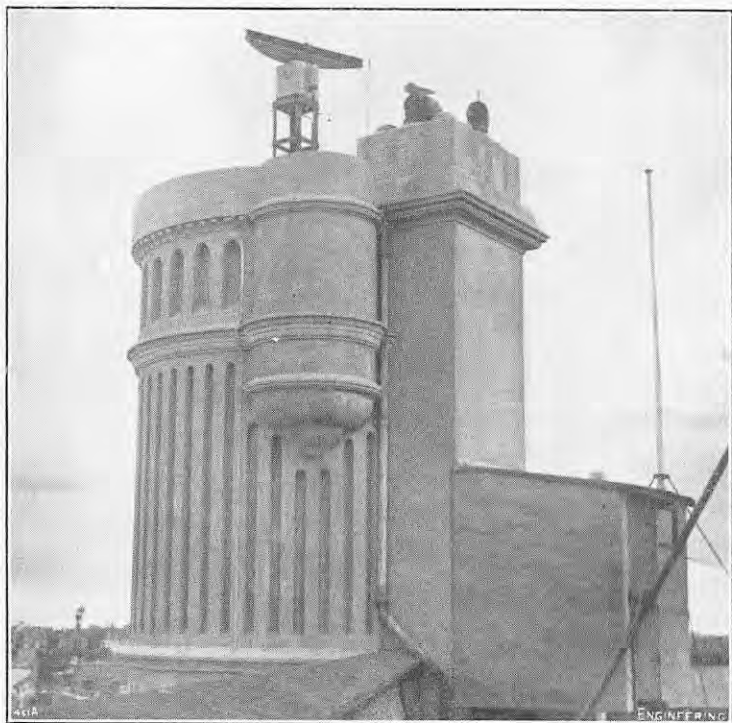
FIG. 1. SCANNER ON TOP OF PALACE HOTEL.
