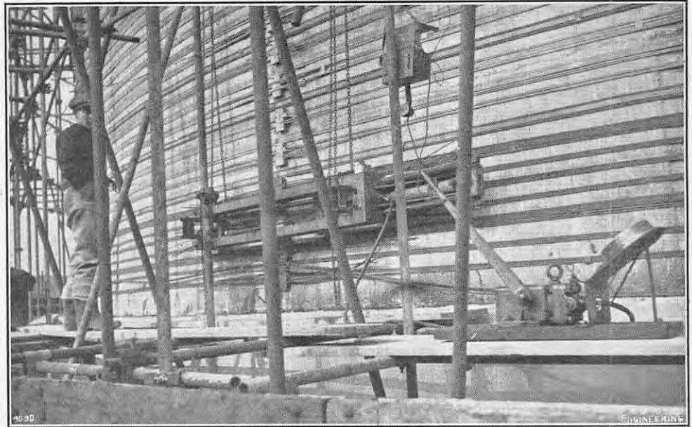
FIG. 2. TENSIONING HORIZONTAL CABLES.
