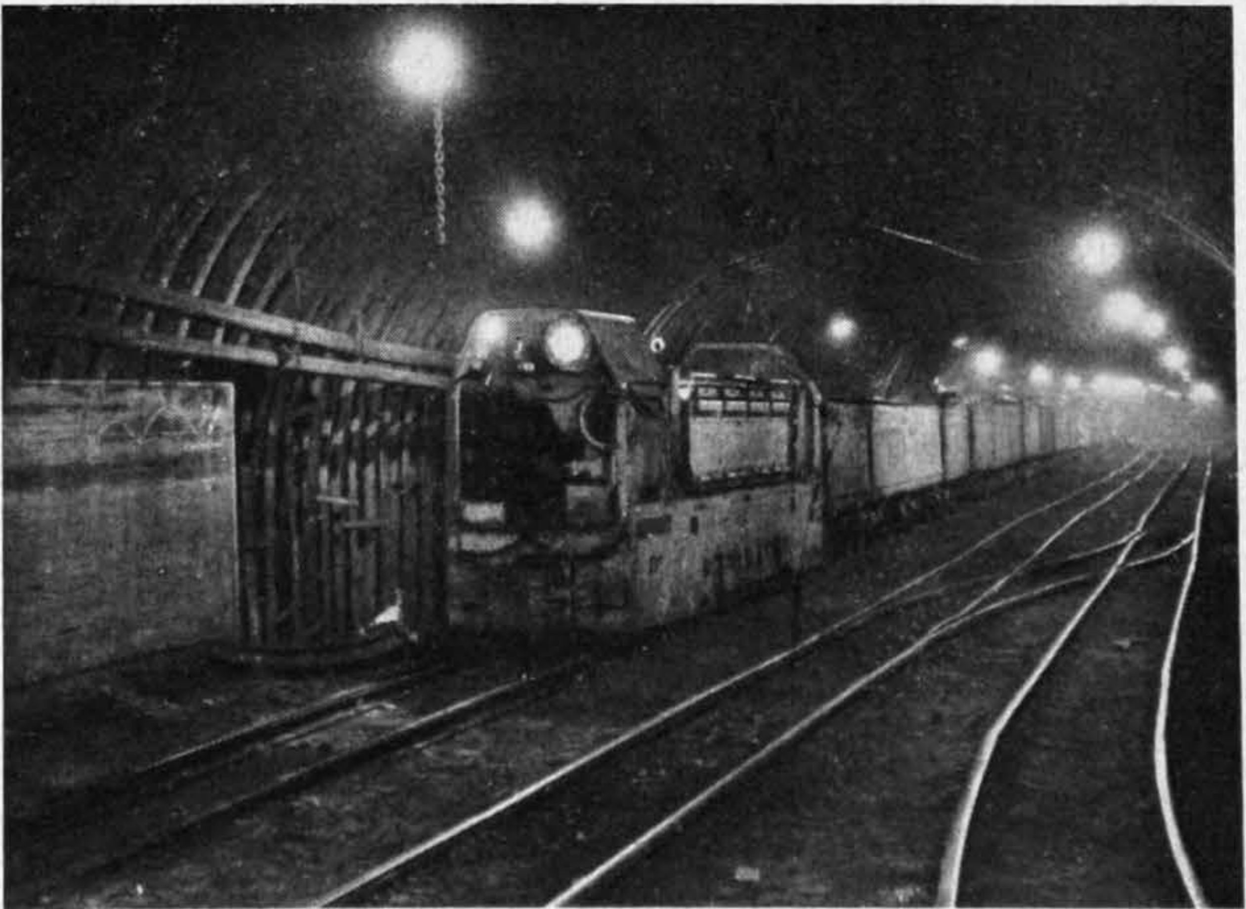
Train of loaded cars arriving at Hawthorn shaft
