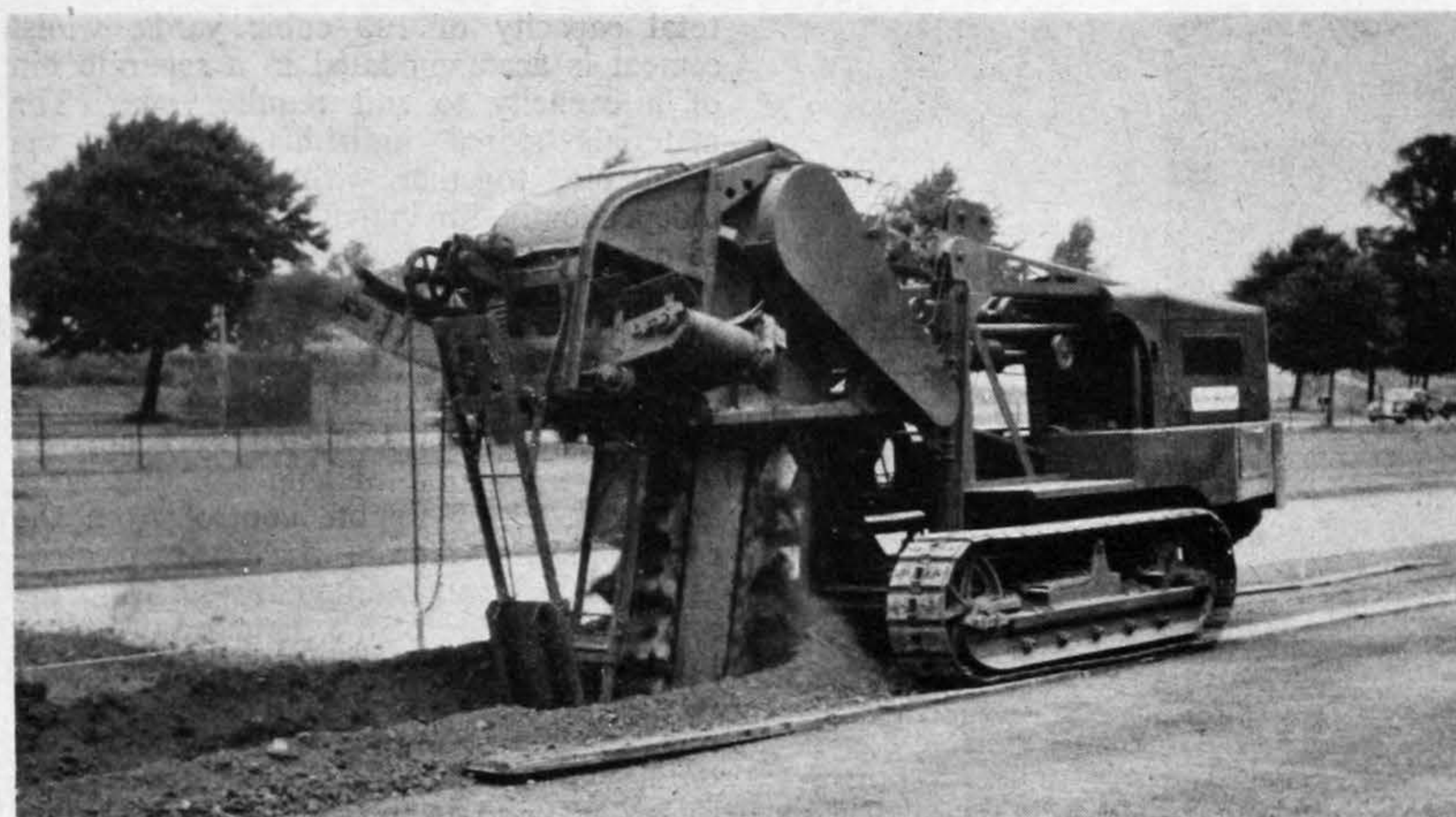
Ditching machine for trenches from 18in to 30in wide and 5ft 6in deep—Barber-Greene Olding
