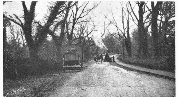
Repairing the road near Carlrow for the Gordon-Bennett race.
