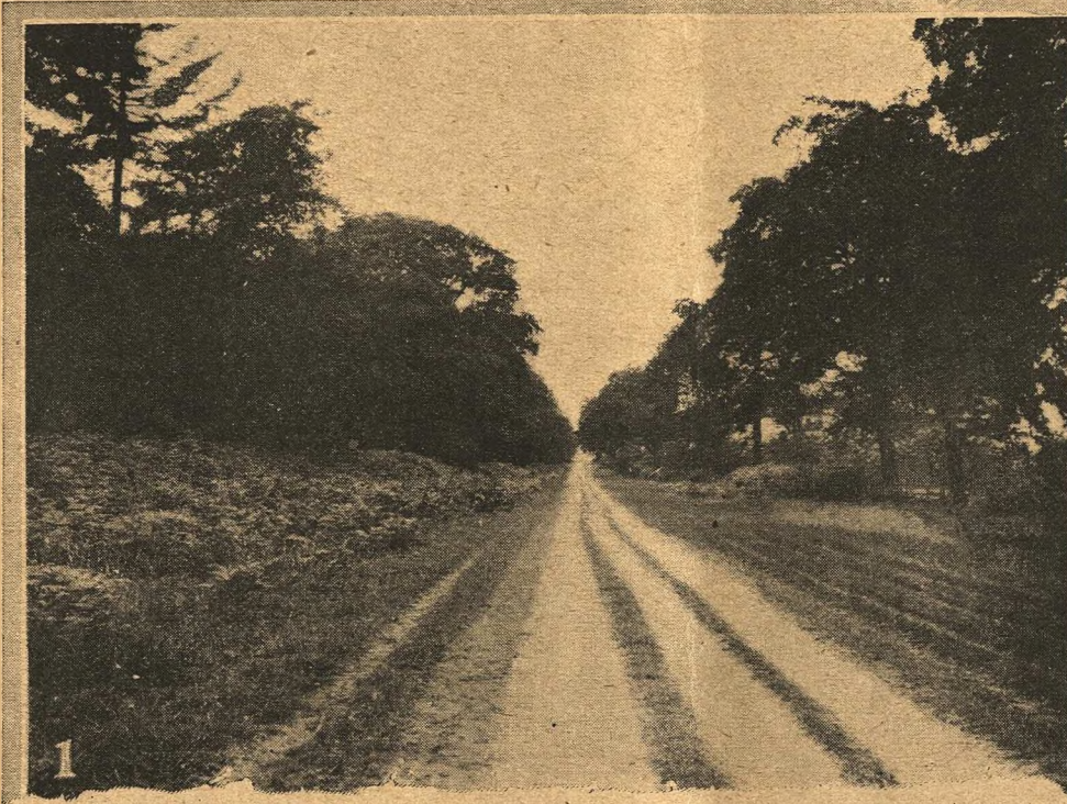
(1) An uneven and grass-grown stretch breaking the continuity of an important link defect—a length of greenway that only needs metalling to join up two useful for want of
