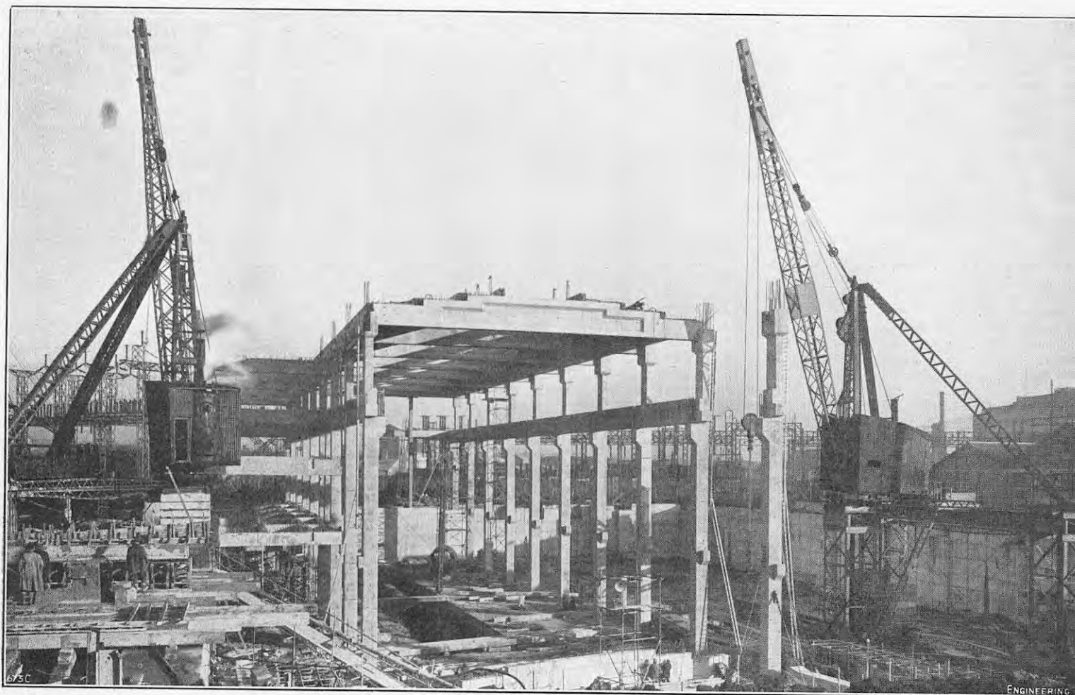
FIG. 3. ERECTING PRE-CAST CONCRETE UNITS OF TURBINE HOUSE; JANUARY 1, 1952.
