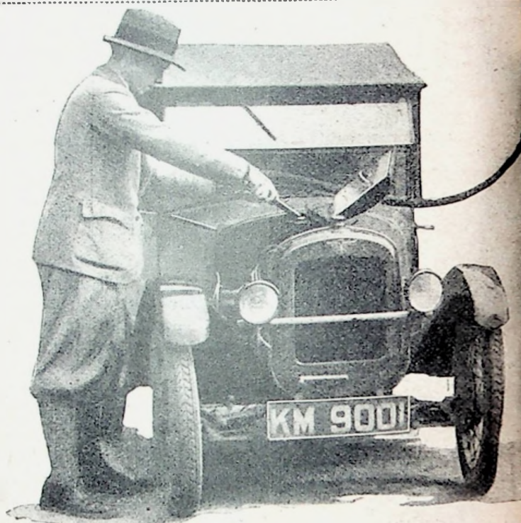
When filling from a pump take care to drain the last drop of petrol from the pipe—they make a big difference to the annual fuel bill.
