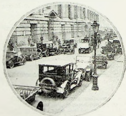
Quarter Day; a photograph outside County Hall, London, on March 25th.
