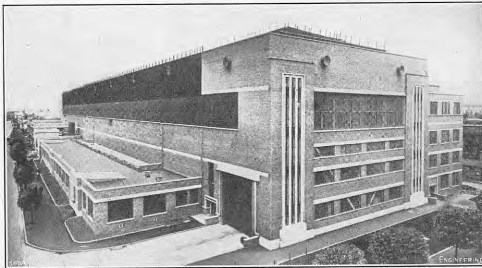
FIG. 1. GENERAL VIEW OF NEW WORKS.
