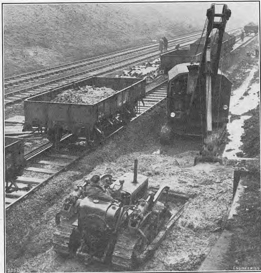
FIG. 4. REMOVAL OF SLURRY FROM WATER-LOGGED FORMATION.
