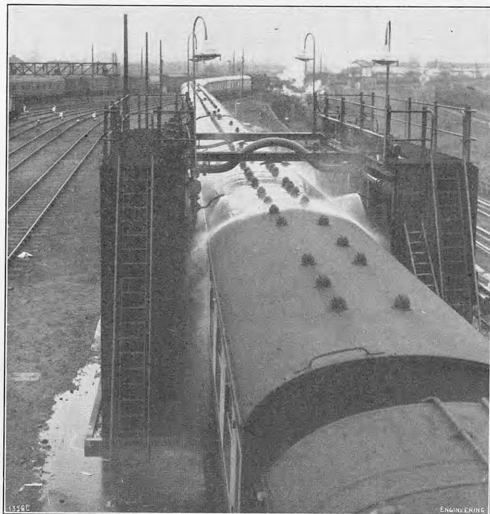
FIG. 3. CARRIAGES PASSING THROUGH WASHING PLANT.
